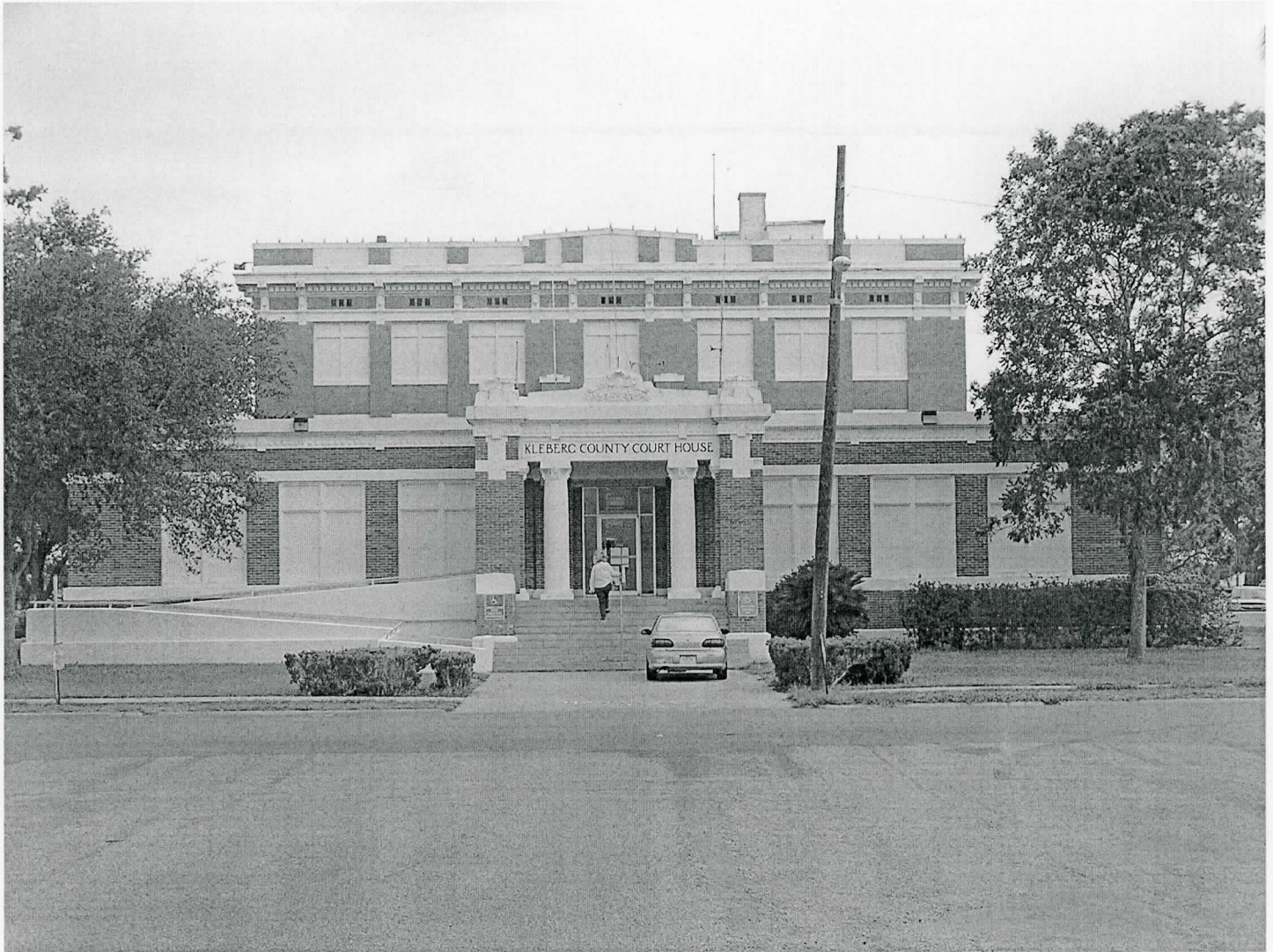
Photo 4. East elevation, camera facing west
