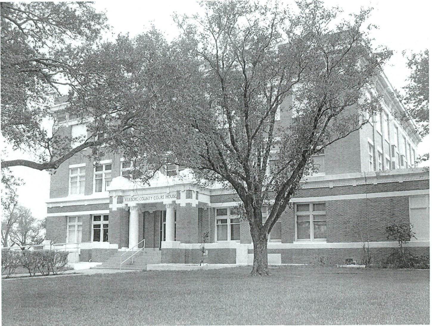
Photo 3. Southeast oblique, camera facing northwest
