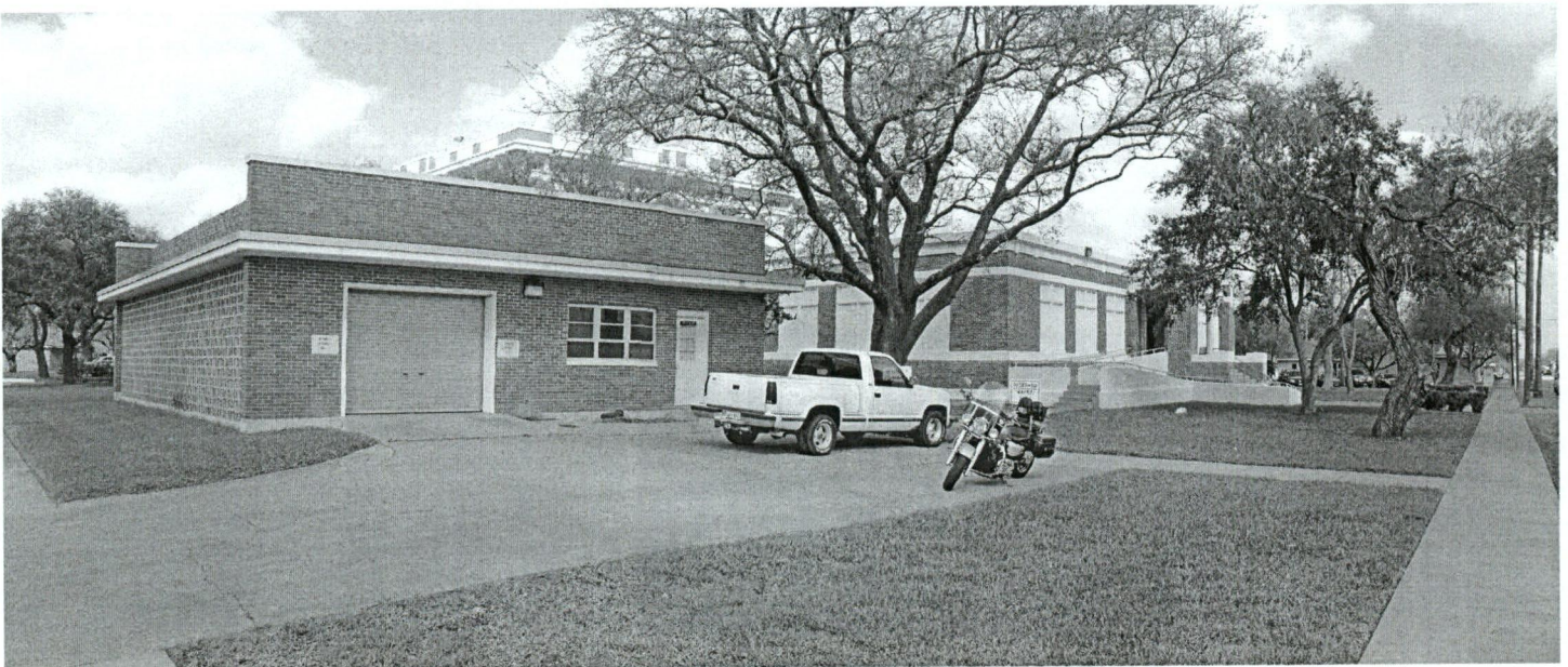
Maintenance and mechanical building, noncontributing.
