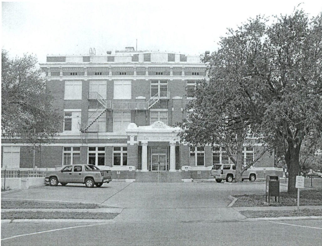
Photo 6. North elevation, camera facing south
