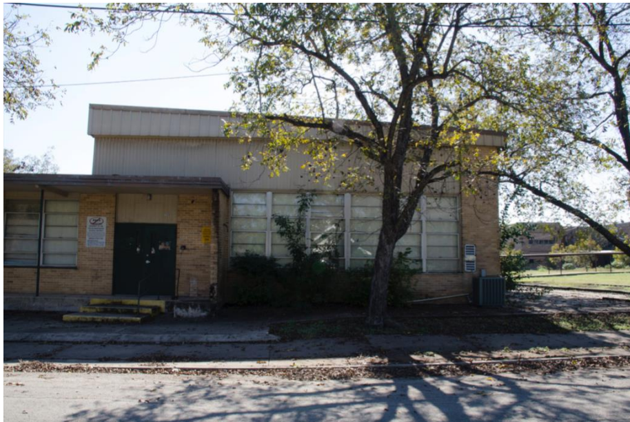
Photo 30: North elevation of junior high, looking south
