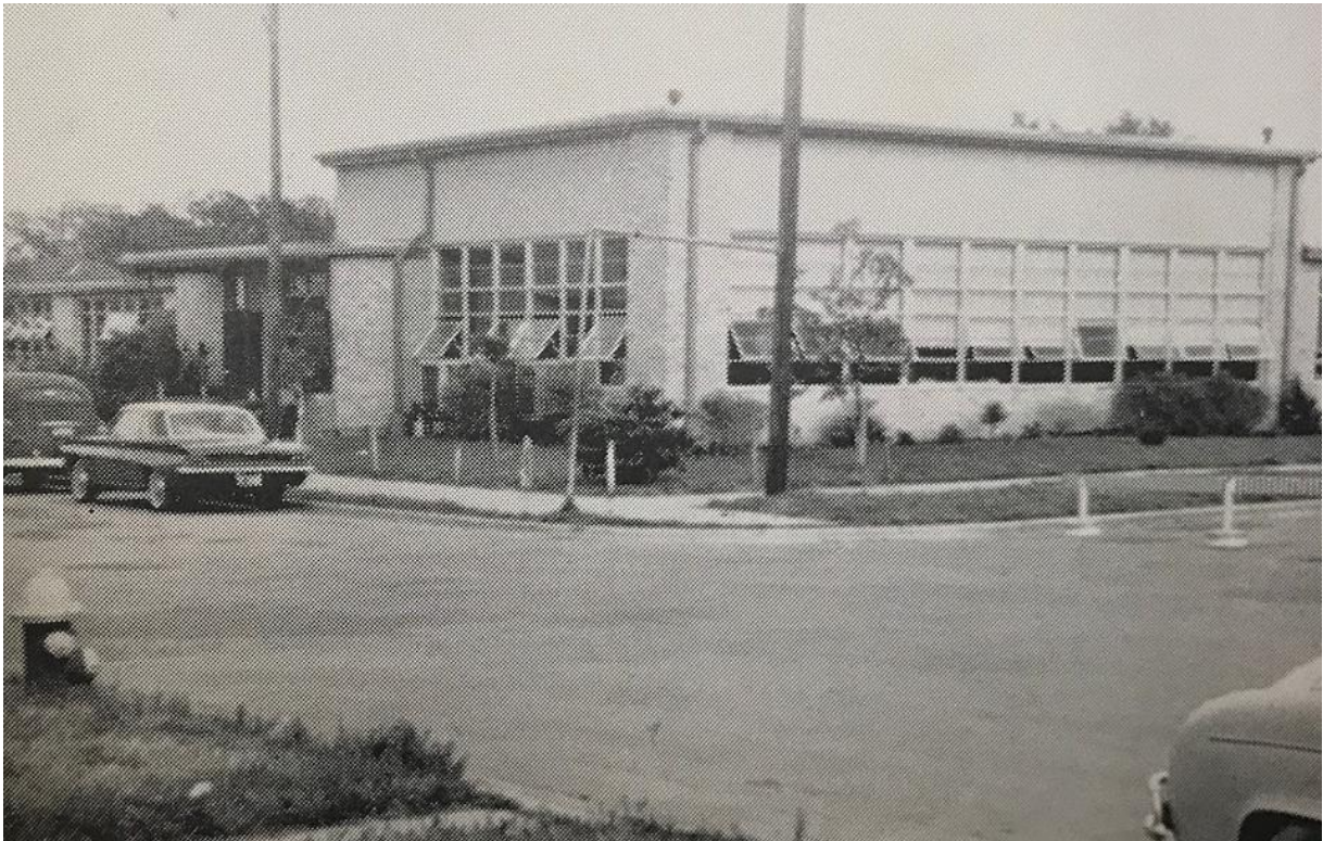
Figure 9: Junior High Building, 1959. Image from the Taylor High School yearbook, housed at the Taylor Public Library
