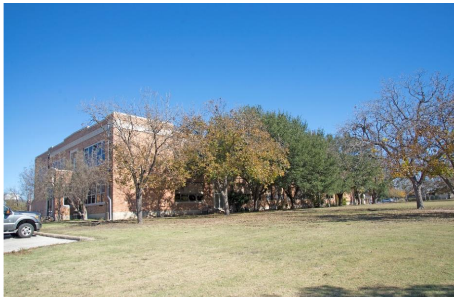
Photo 3: South and west elevation, looking northeast
