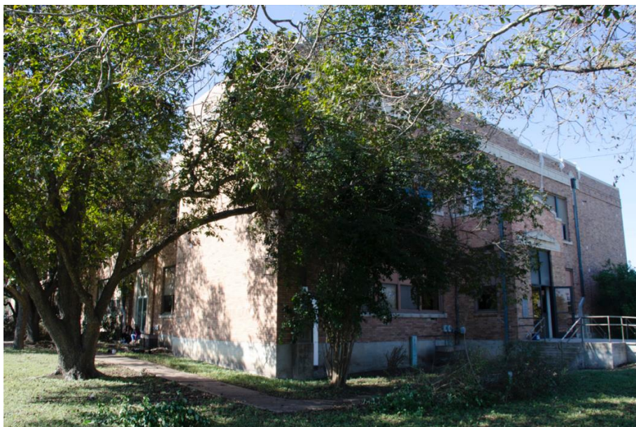
Photo 6: East and south elevations, looking northwest
