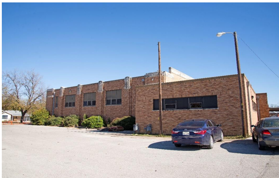
Photo 24: West elevation of gymnasium, looking east
