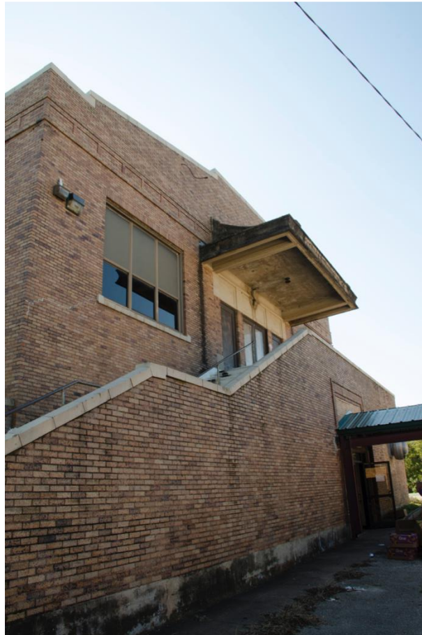
Photo 8: North elevation of auditorium, looking southwest
