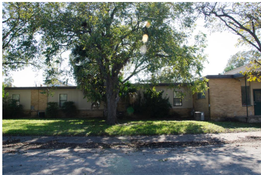
Photo 31: North elevation of junior high, looking south
