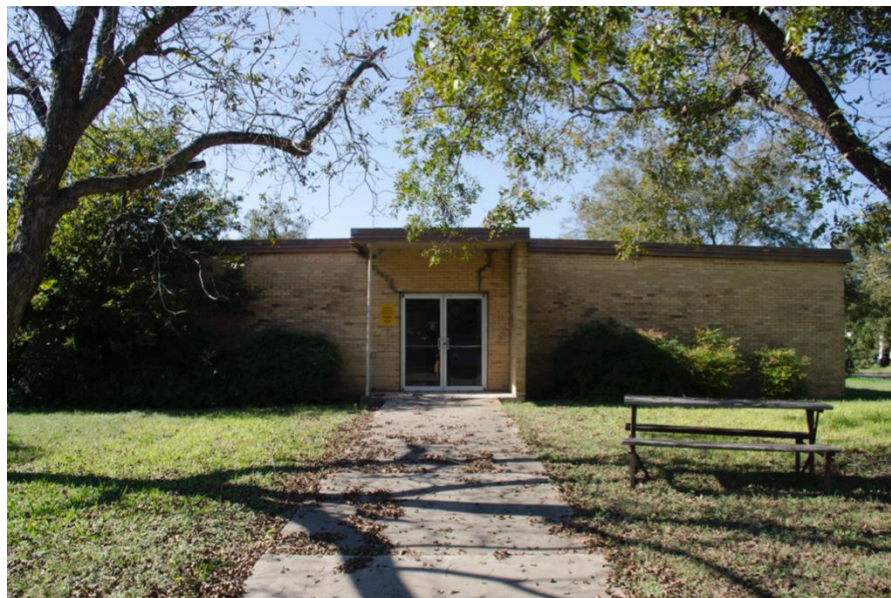
Photo 32: East elevation of junior high, looking west
