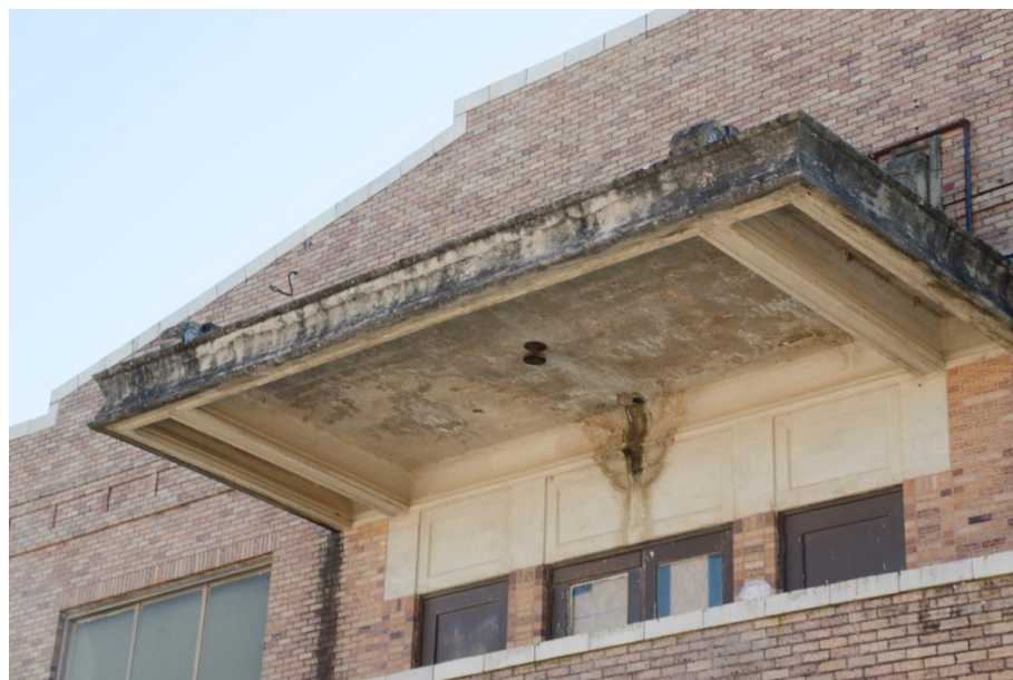
Photo 10: North elevation of auditorium, detail of entrance, looking south
