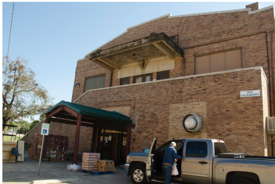
Photo 9: North elevation of auditorium, looking south
