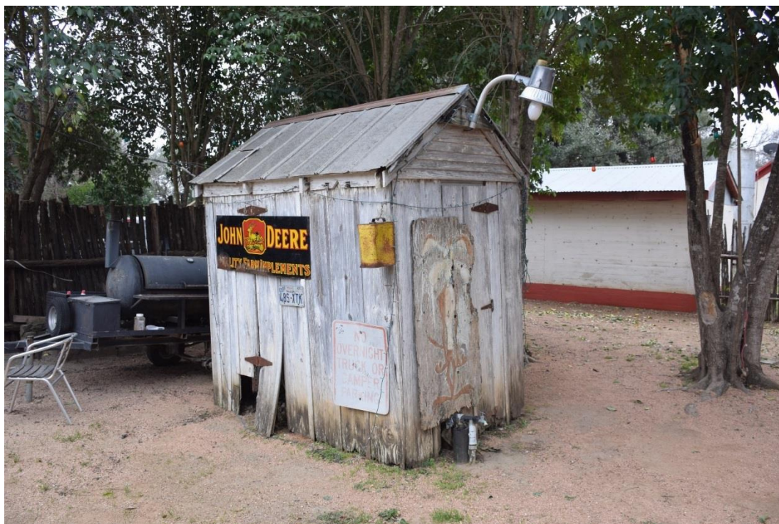
Photo 33. Oblique view of water pump shed (Resource #3), view facing south.
