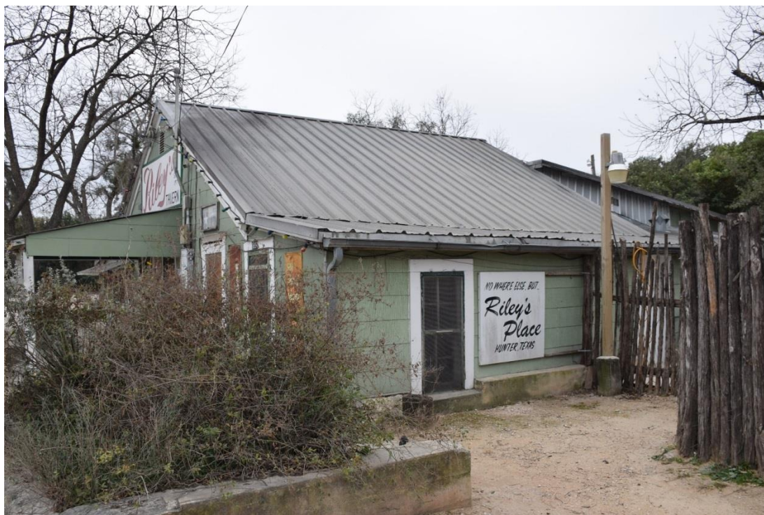
Photo 5. Oblique view of Riley's Tavern (Resource #1), view facing south.
