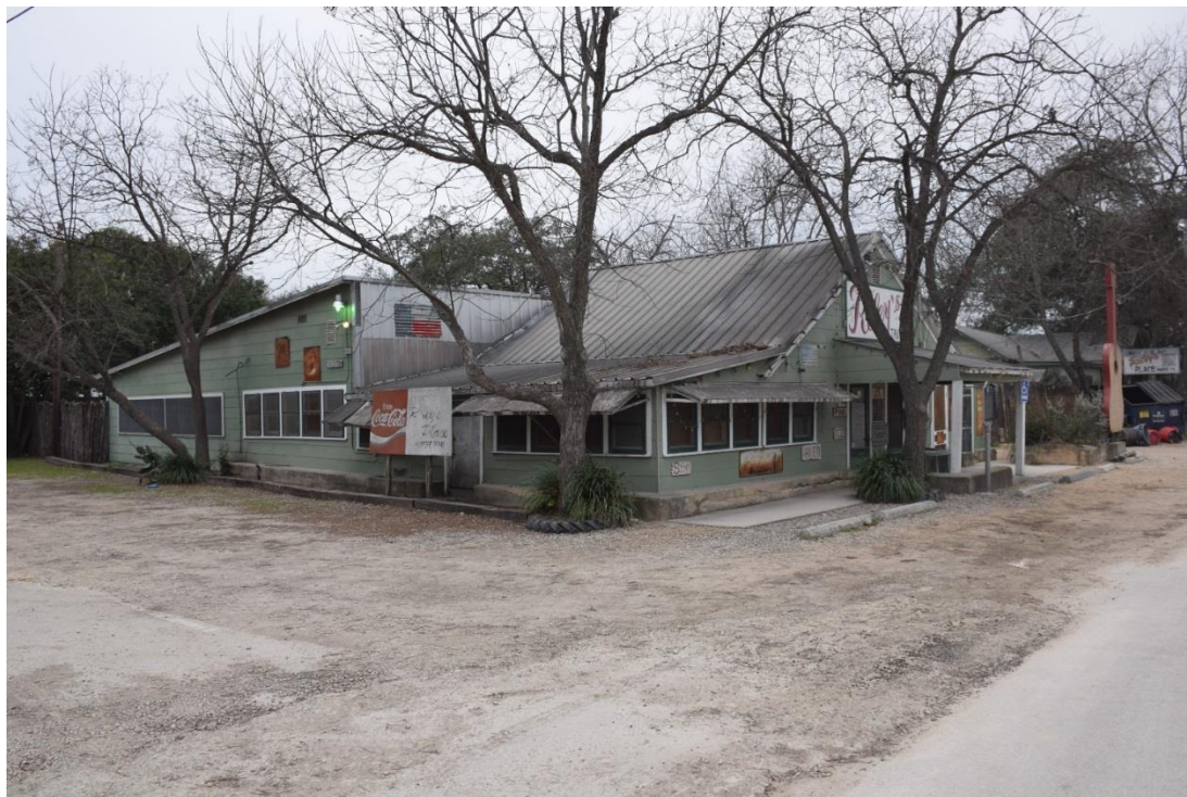
Photo 3. Oblique view of Riley's Tavern (Resource #1), view facing west.
