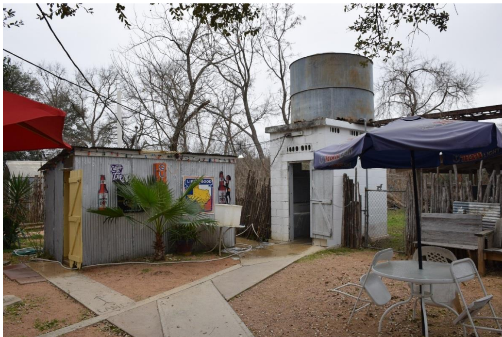
Photo 32. Oblique view of bathroom shed (Resource #2), view facing southwest.
