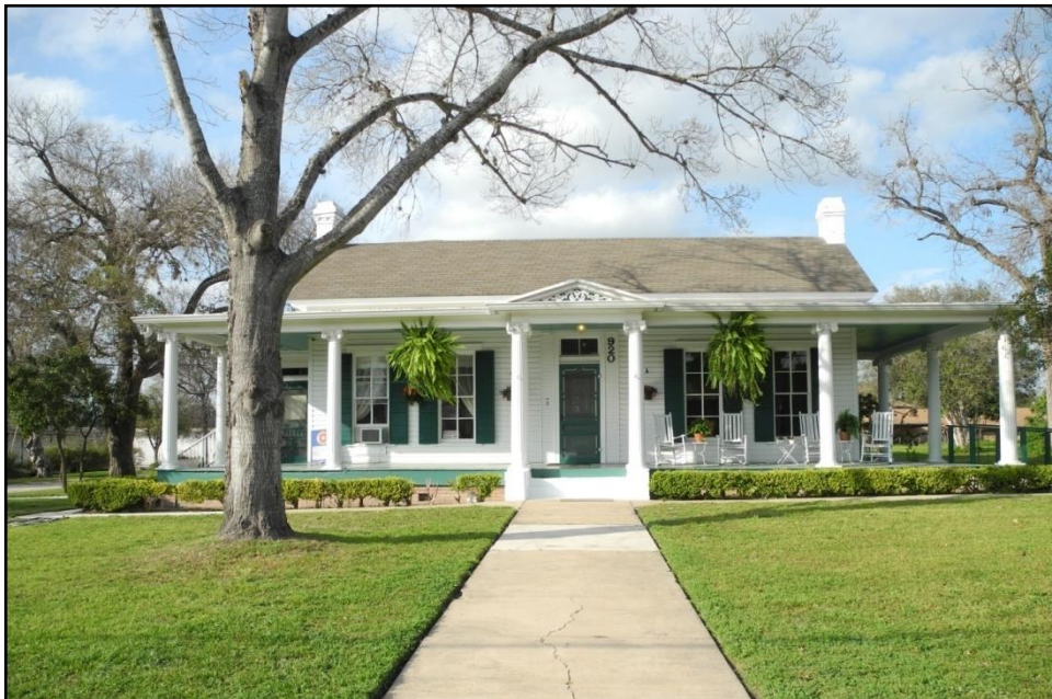
PHOTO 1: King-Woods House, south elevation, facing north (February 1, 2017).
