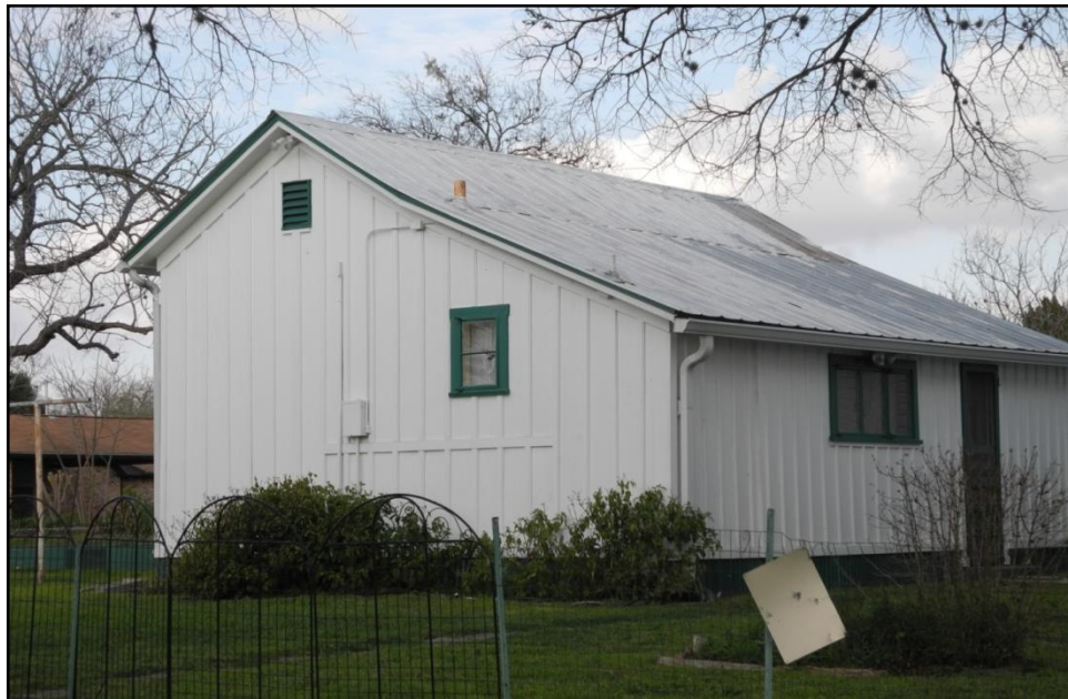
PHOTO 15: King-Woods Kitchen/Smokehouse, east and north elevations, facing southwest (February 1, 2017).
