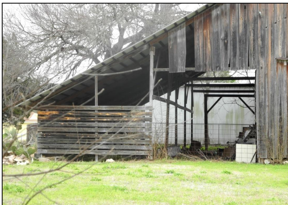
PHOTO 12: King-Woods Multi-purpose Barn, horse stalls, west elevation, facing east/northeast (December 10, 2016).
