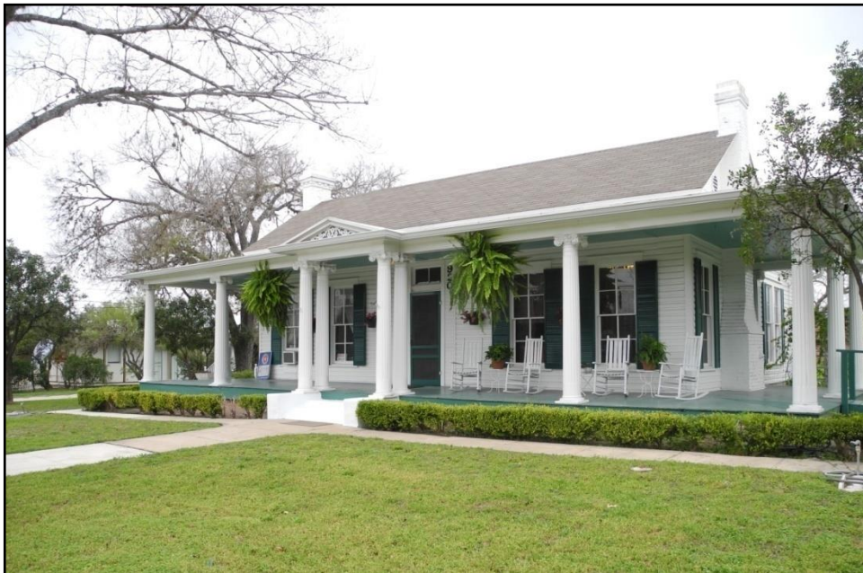
PHOTO 3: King-Woods House, south and east elevations, facing northwest (February 1, 2017).
