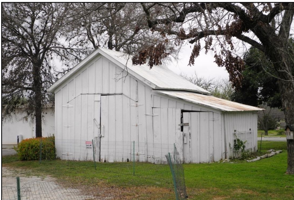
PHOTO 14: King-Woods Buggy House, south and east elevations, facing north/northwest (February 1, 2017).
