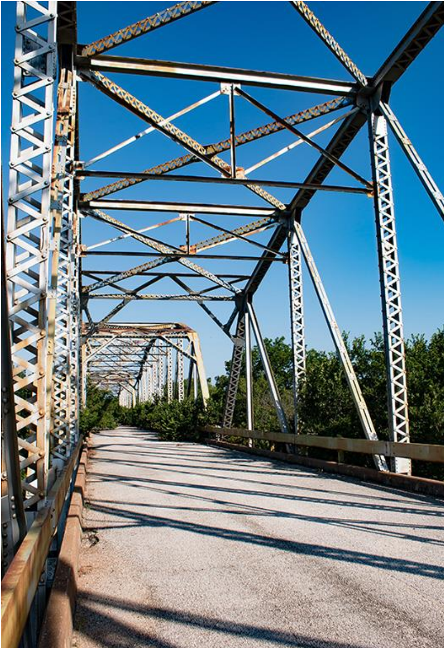
Photo 2 Facing west from center span
