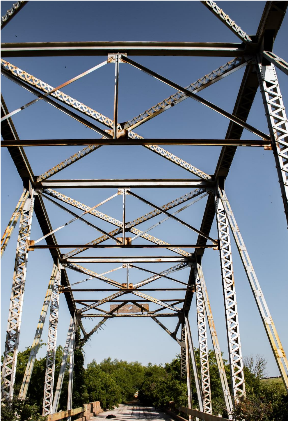
Photo 7 Easternmost span, facing west towards approach spans
