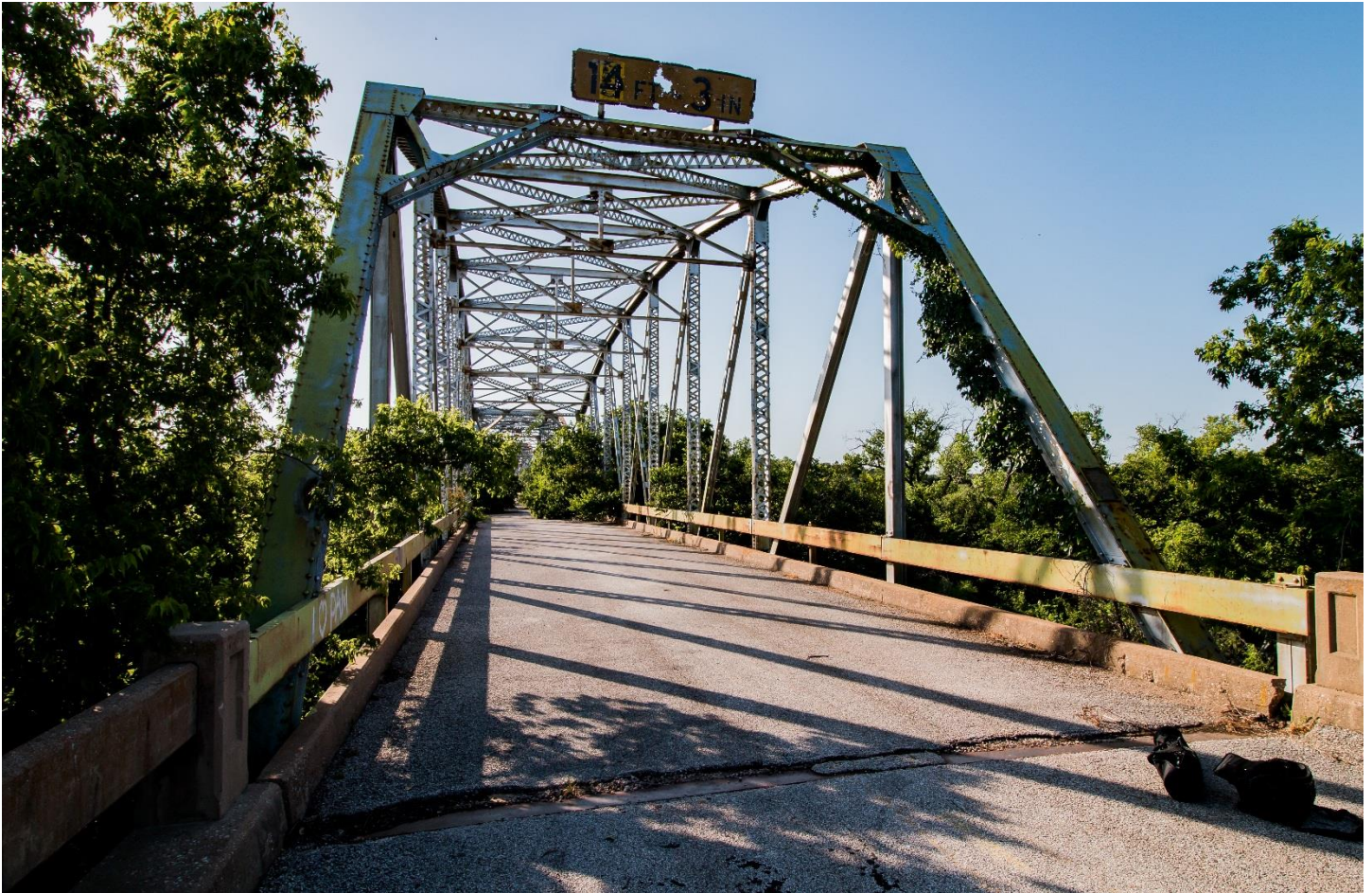
Photo 3 West end, camera facing east
