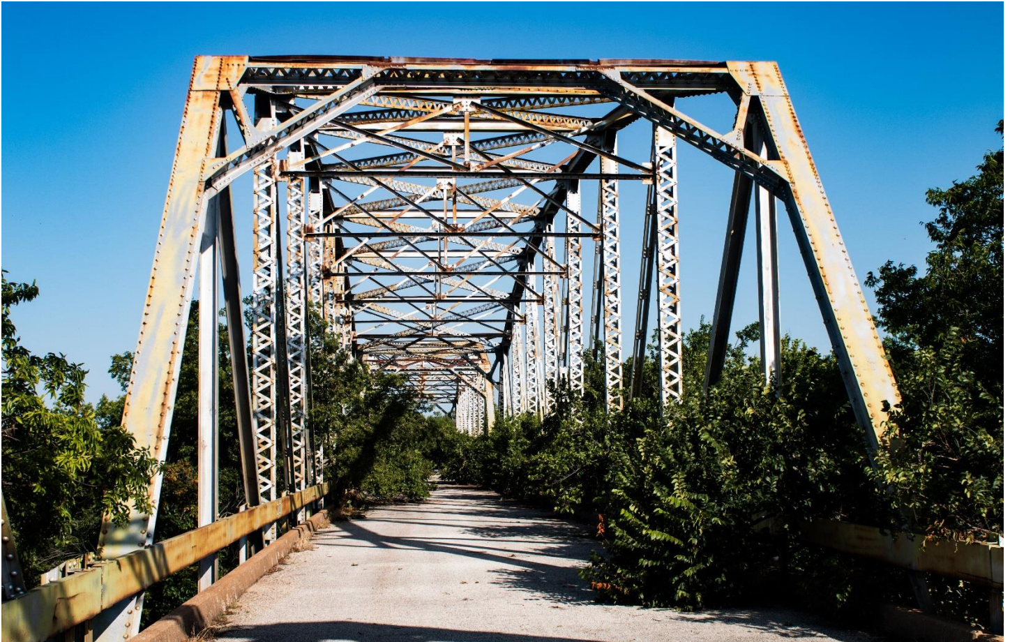
Photo 4 Facing west from center span
