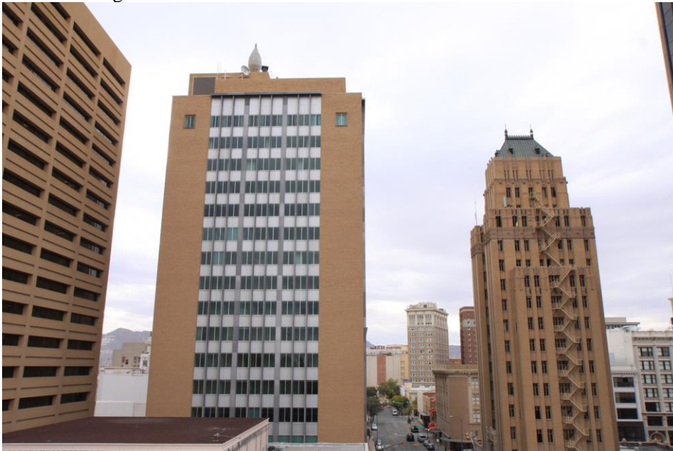
Photo 3 East Façade Camera facing west
