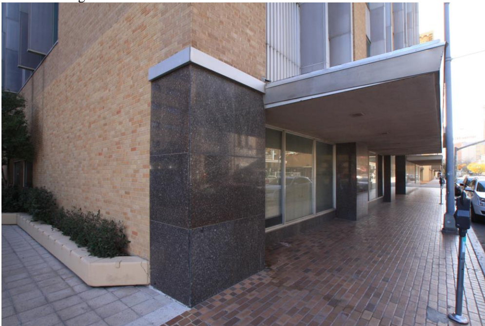
Photo 11 Ground floor at northeast corner Camera facing southwest
