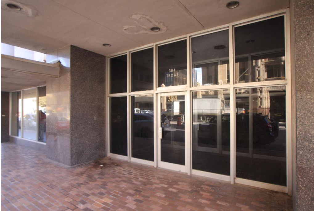
Photo 10 Main Entry, north side Camera facing southeast
