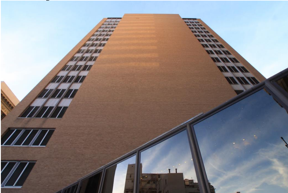
Photo 8 South elevation, looking up Camera facing north
