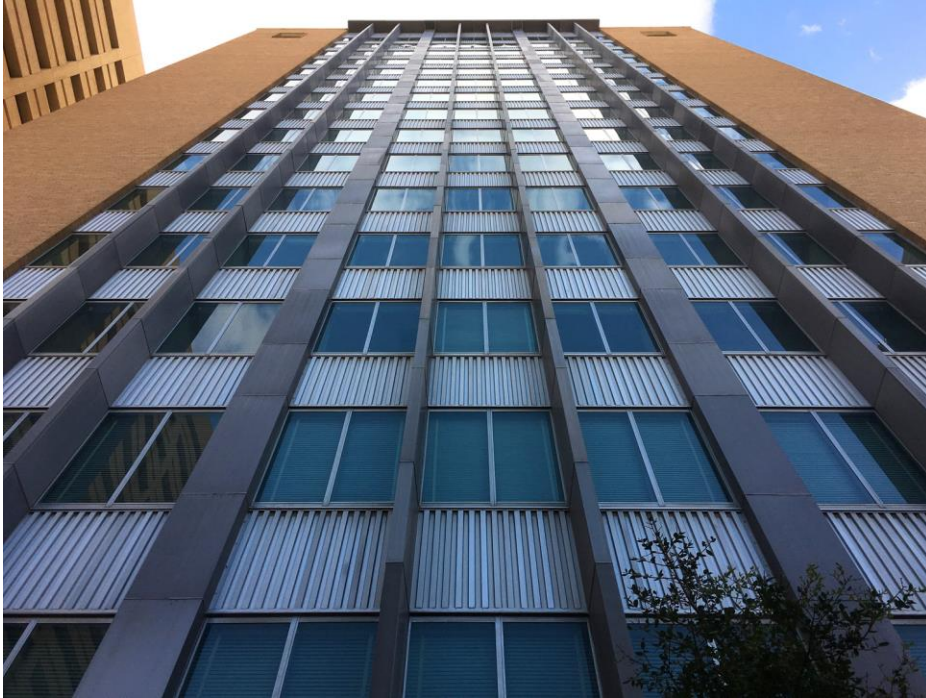
Photo 6 East Façade, looking up Camera facing west
