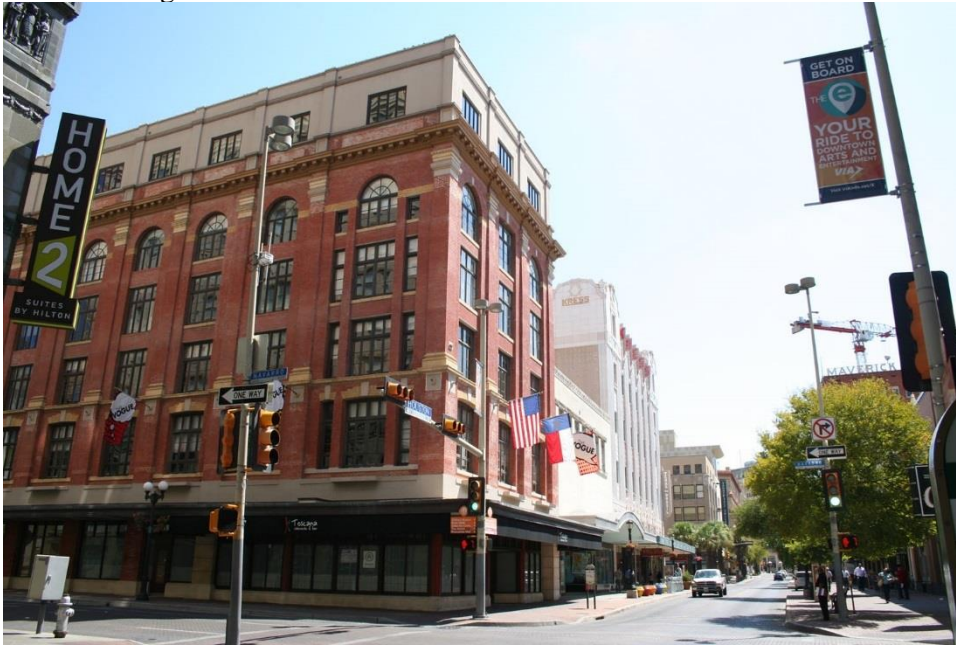
Photo 75 300 Block E Houston, with Peck / Vogue Building Camera facing NE
