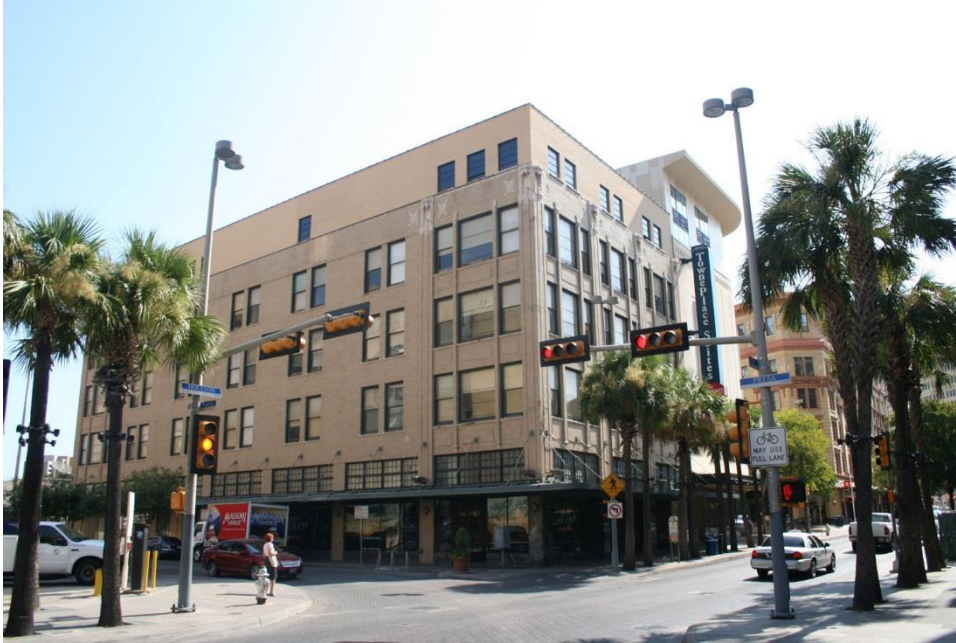
Photo 13 401 E Houston, Burns Building Camera facing NE
