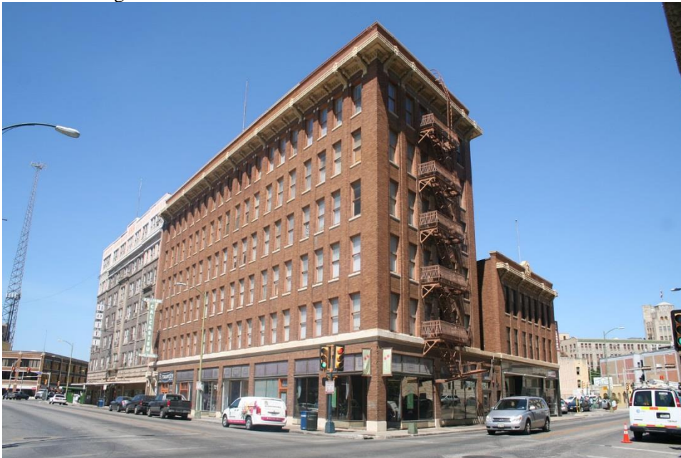
Photo 14 214 Broadway, Calcasieu Building Camera facing NE
