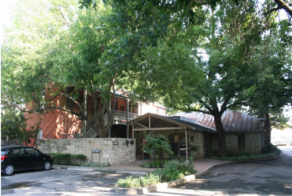
Photo 1 214 W Salinas, Garcia-Garza House Camera facing NW
