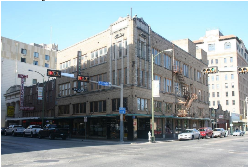
Photo 70 Broadway Street, with Goggan Building Camera facing SW
