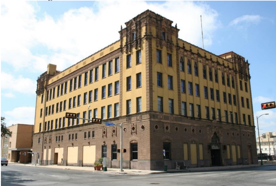
Photo 27 420 Broadway, San Antonio Light Building Camera facing S
