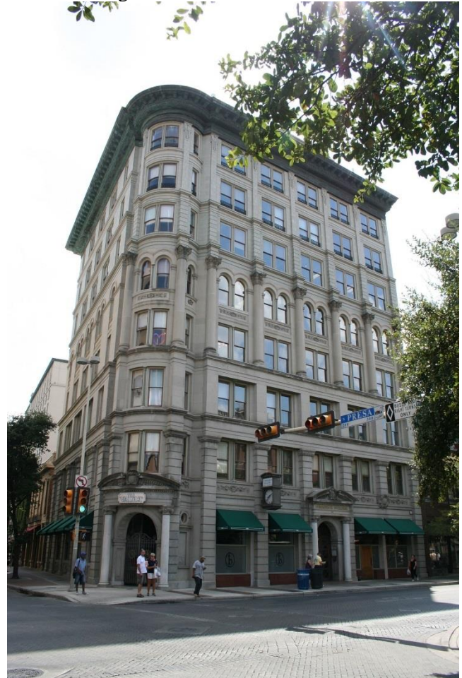
Photo 12 314/316 E Commerce, (Old) Alamo National Bank Building Camera facing SW
