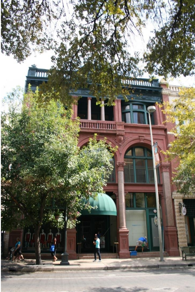
Photo 9 309 E Commerce, Staacke Brothers Building Camera facing N
