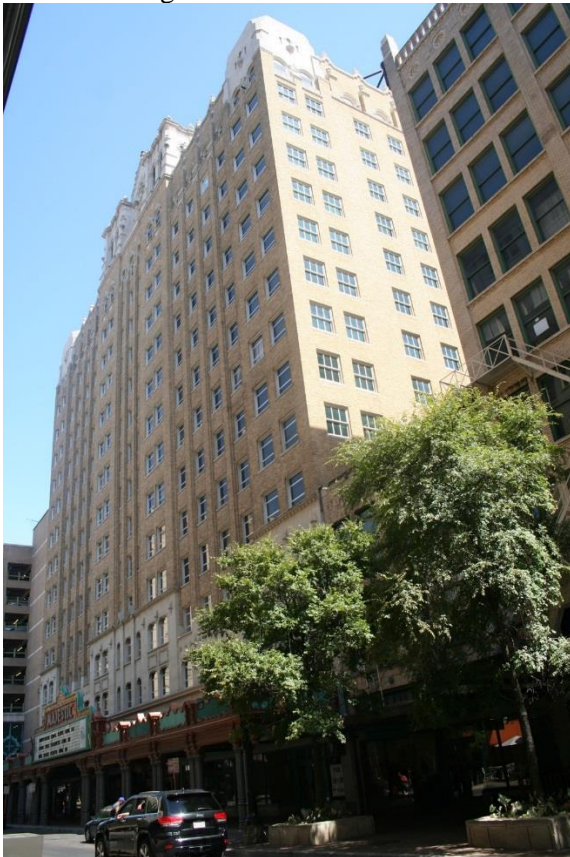
Photo 18 216/230 E Houston, The Majestic Theater Camera facing SE
