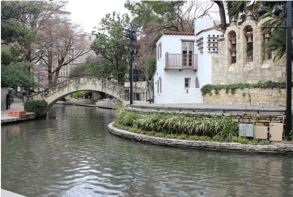
Photo 61 Arneson Theater Stage house Camera facing W
