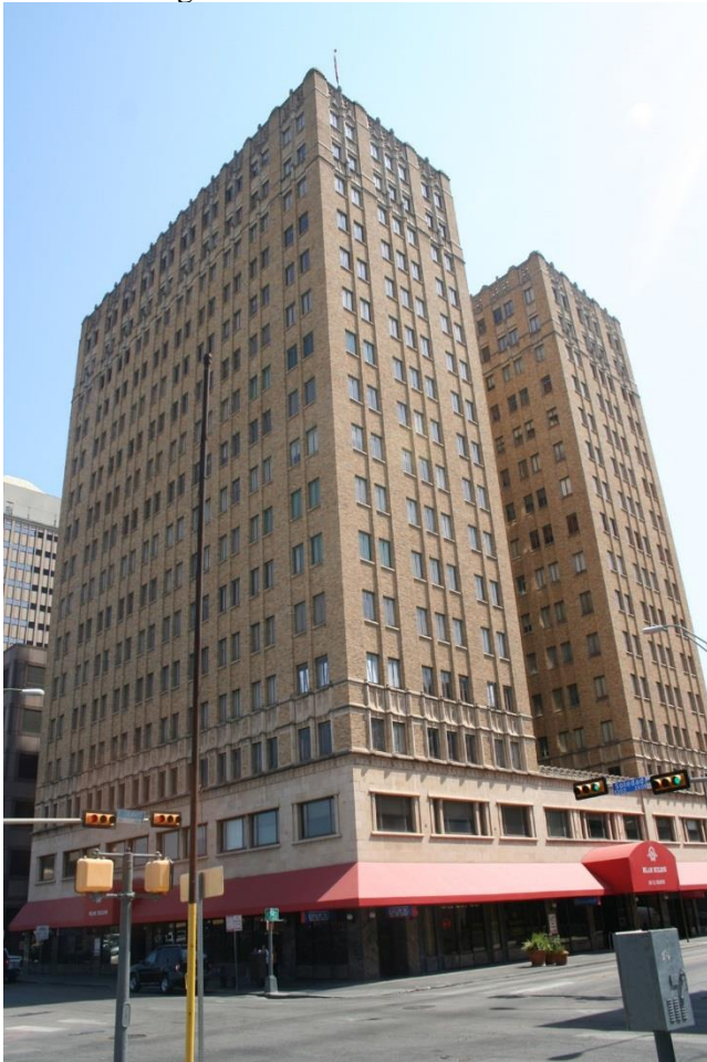
Photo 25 115 E Travis, Milam Building Camera facing NE
