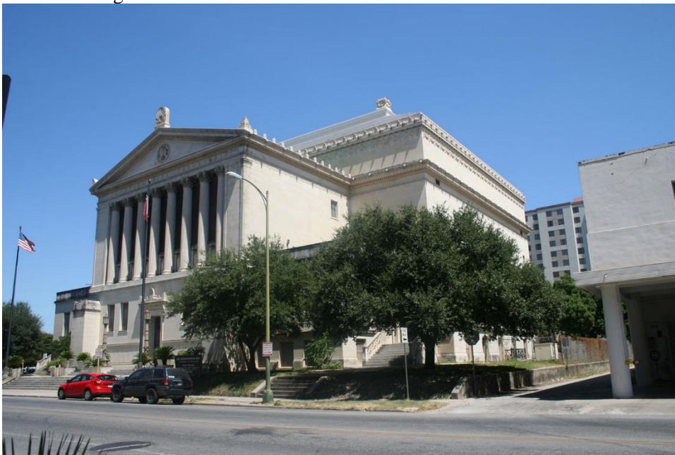
Photo 4 308 Ave E, Scottish Rite Cathedral Camera facing NE
