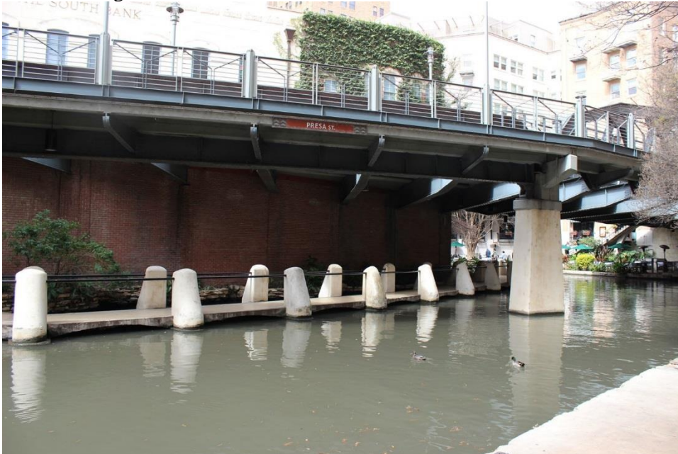
Photo 51 Block 14 (Presa N Street Bridge S21 to Crockett E Bridge S11) Floating walk Camera facing W
