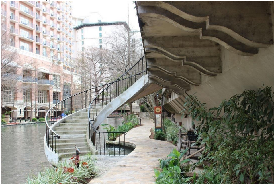
Photo 62 Block 19 (Mill Bridge S17 to St. Mary's S Street Bridge S27) Curved midblock stairway Camera facing E
