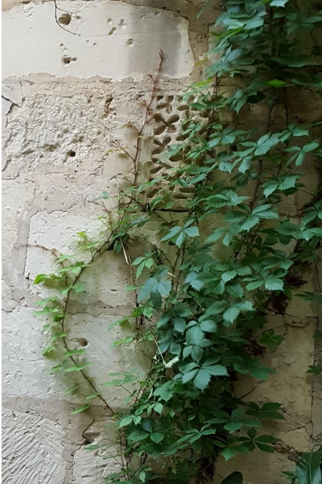
Photo 45 Block 10 (Houston Bridge S12 to Upper Flood Gate) Recycled walls Camera facing W
