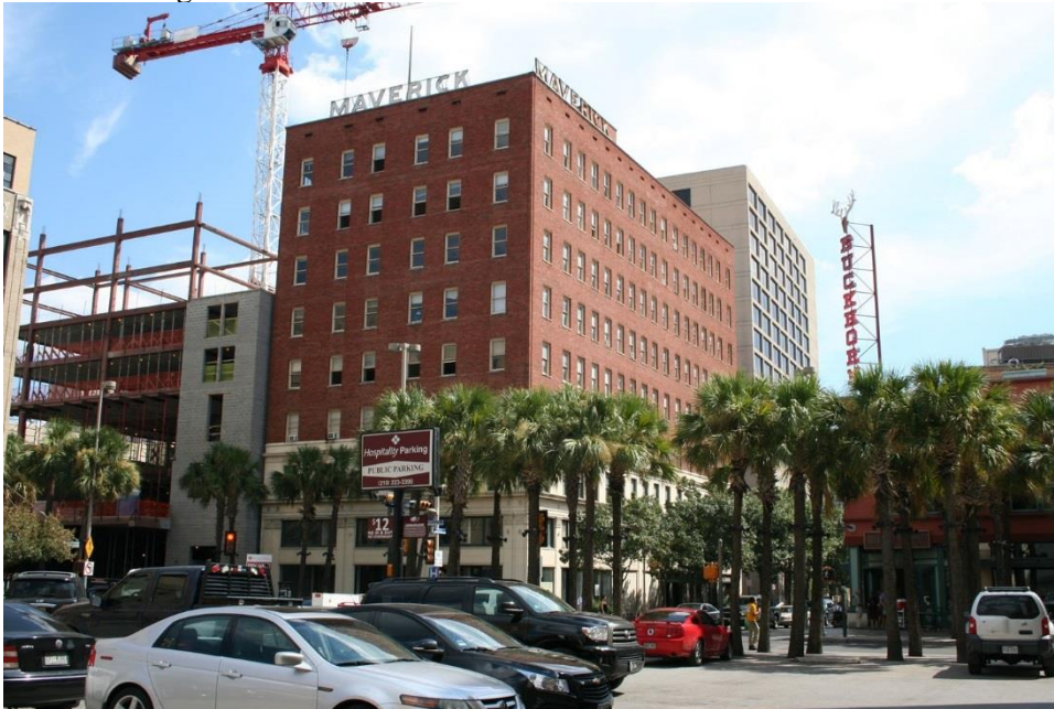
Photo 77 George Maverick Building Camera facing SE
