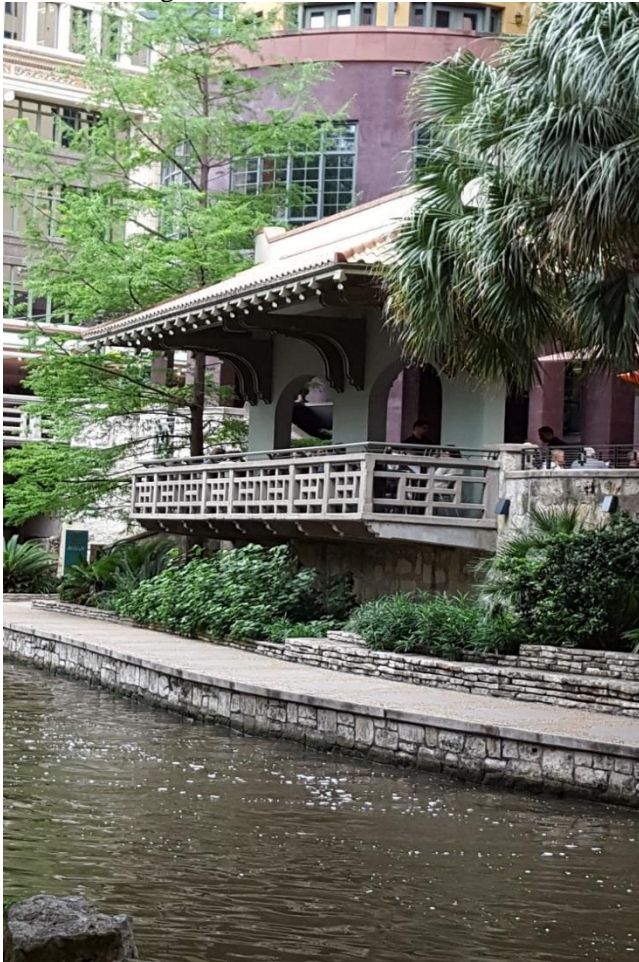
Photo 43 Block 10 (Houston Bridge S12 to Upper Flood Gate) Balcony Camera facing NE
