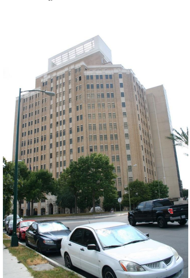
Photo 26 105 Auditorium Circle, Southwestern Bell Building Camera facing SW
