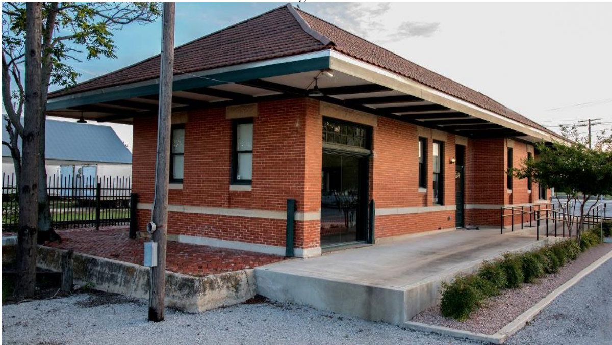
Photo 4: North and east elevations—camera facing southwest
