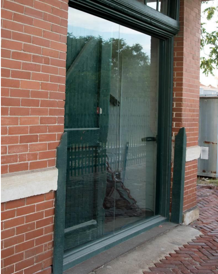
Photo 9: Baggage Room door detail—camera facing north northeast showing door inside fixed glass
