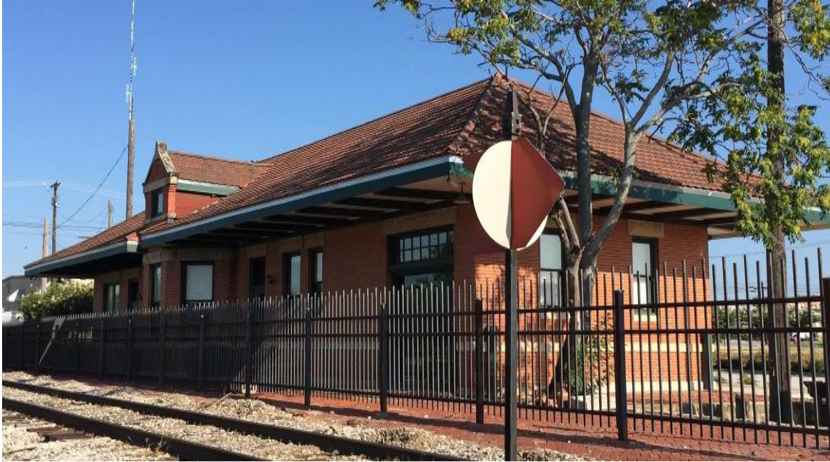
Photo 3: South and east elevations—camera facing northwest, June 10, 2017, Margaret Dudley
