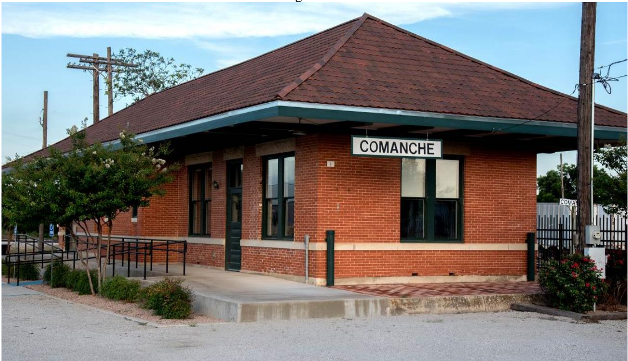
Photo 6: North and west elevations—camera facing southeast
