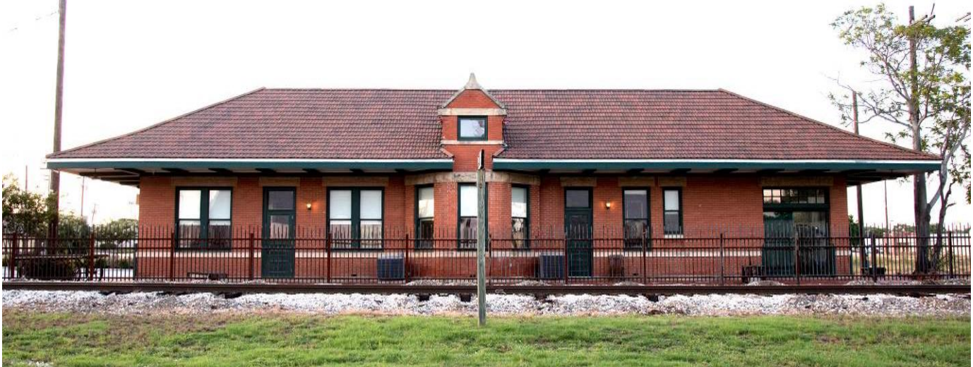
Photo 1: South elevation—camera facing north
