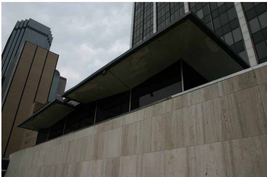
Photo 18 Exterior of glass clerestory and canopy at level 9 North elevation
