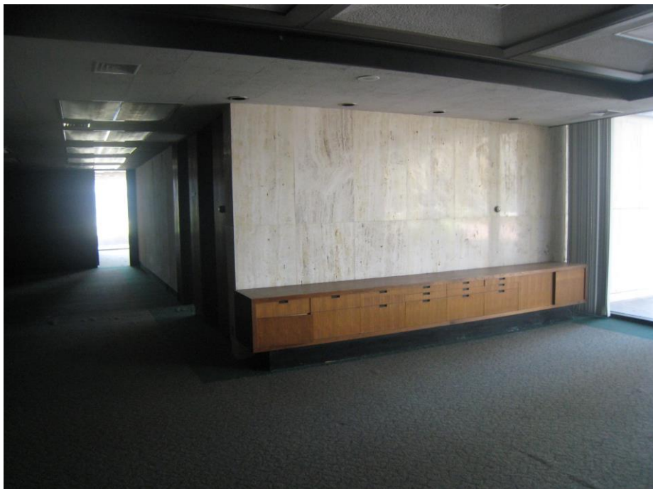
Photo 30 9 th floor main lobby Typical finishes of this area (travertine, teak wood millwork and wall panels)
