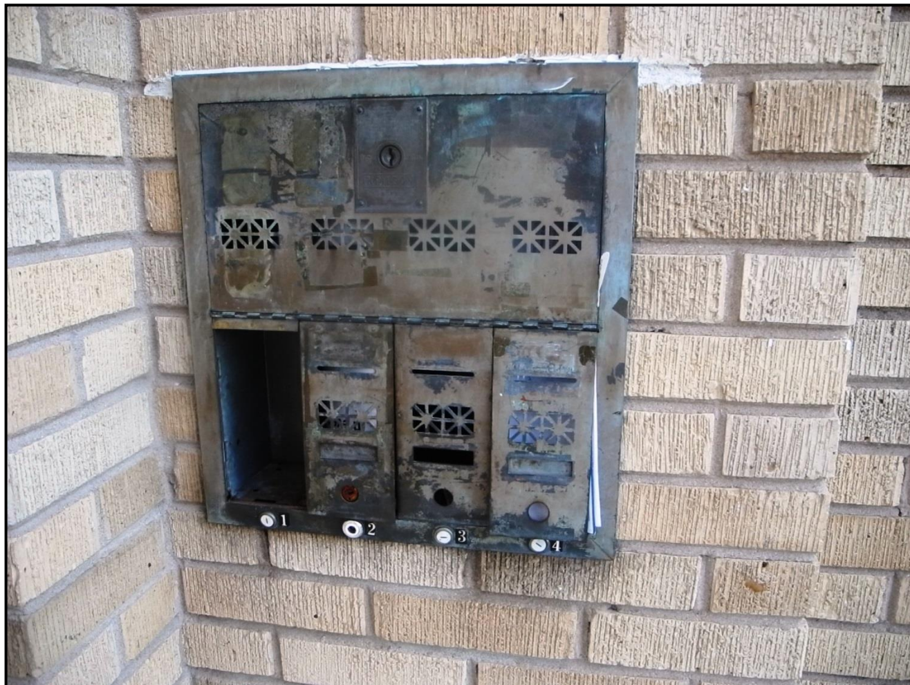
Original Mailboxes – Exterior Entry Wall
