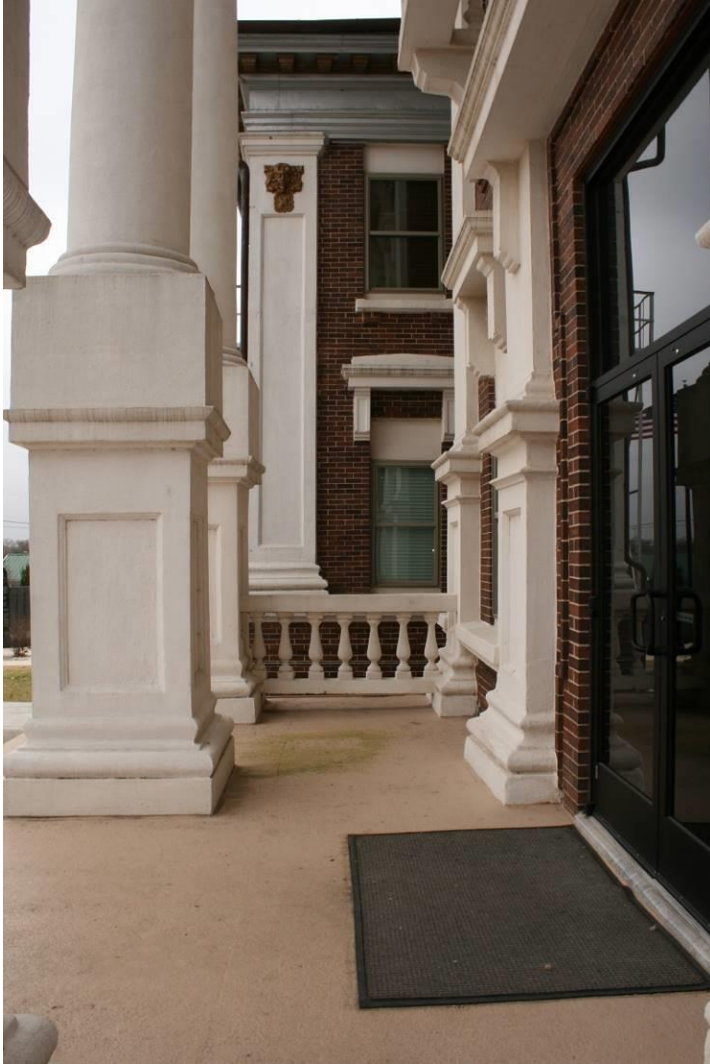
Photo 6: Looking east at details of north porch
