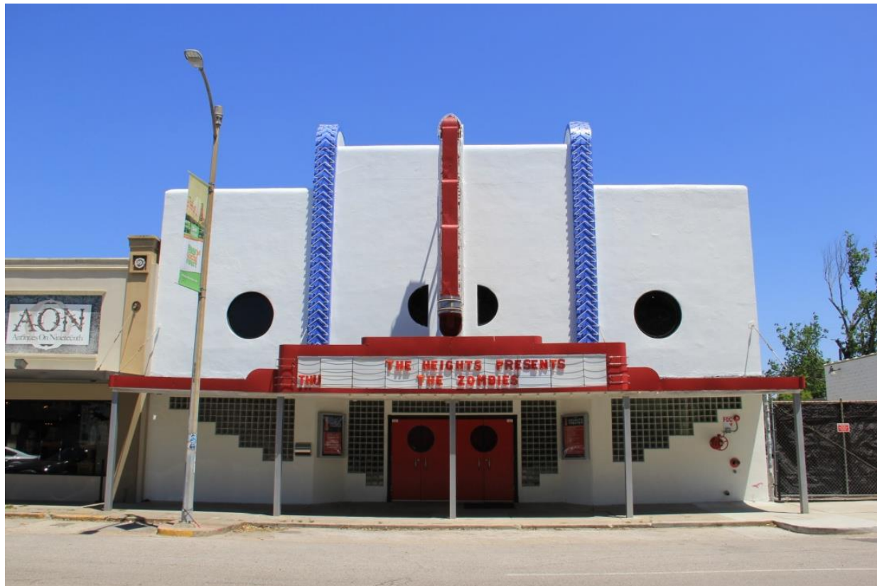
Photo 3: South Facade, looking north, May 5, 2017
