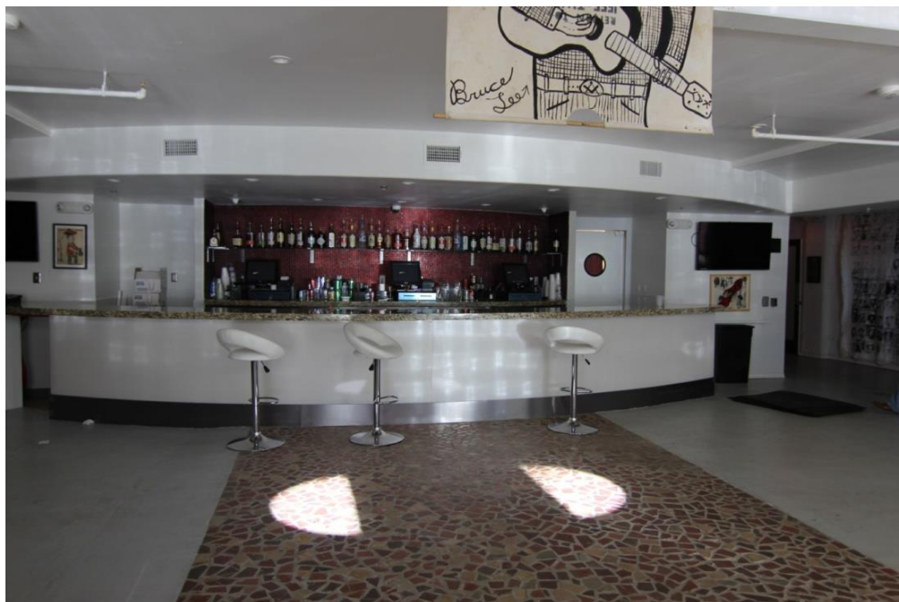
Photo 7: First floor lobby and bar; bar front at center and 'broken' ceramic tile re-laid in new concrete floor, looking north. January 30, 2017
