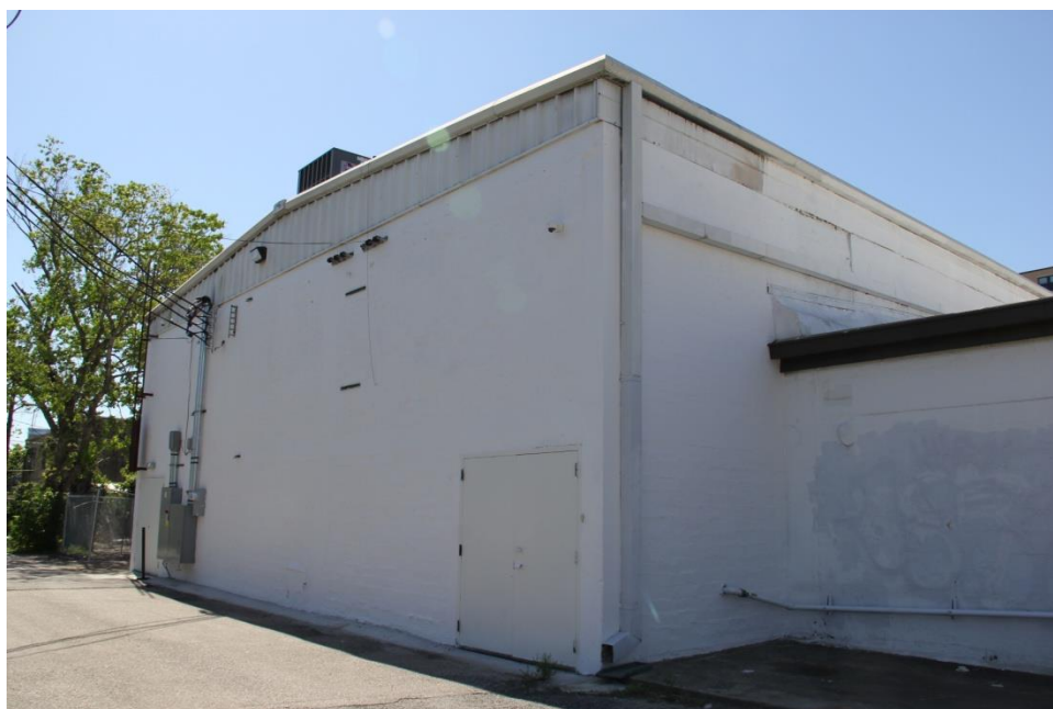
Photo 5: North and partial west (right side) Facades, looking southeast, May 5, 2017
