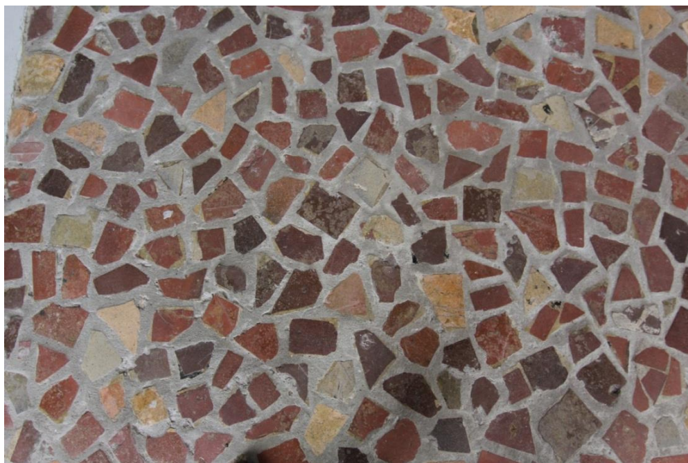
Photo 9: Detail of broken tile re-laid at First Floor Lobby, January 30, 2017
