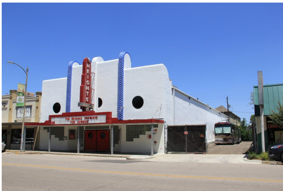
Photo 2: South facade, looking northwest, May 5, 2017
