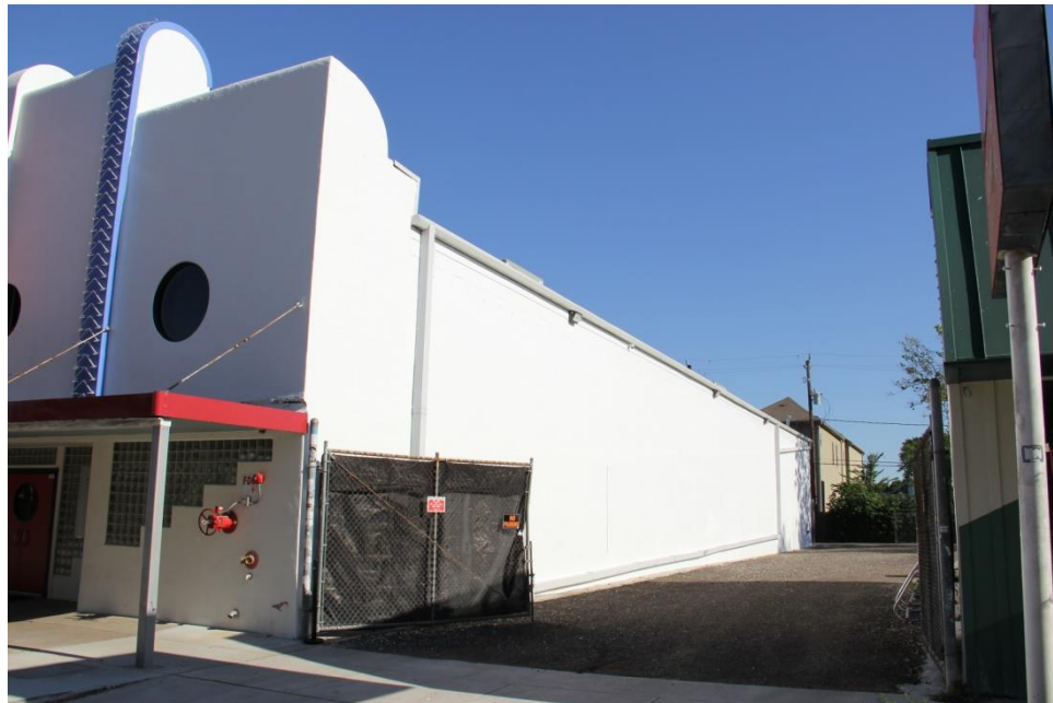
Photo 4: East Facade, looking northwest, May 5, 2017
