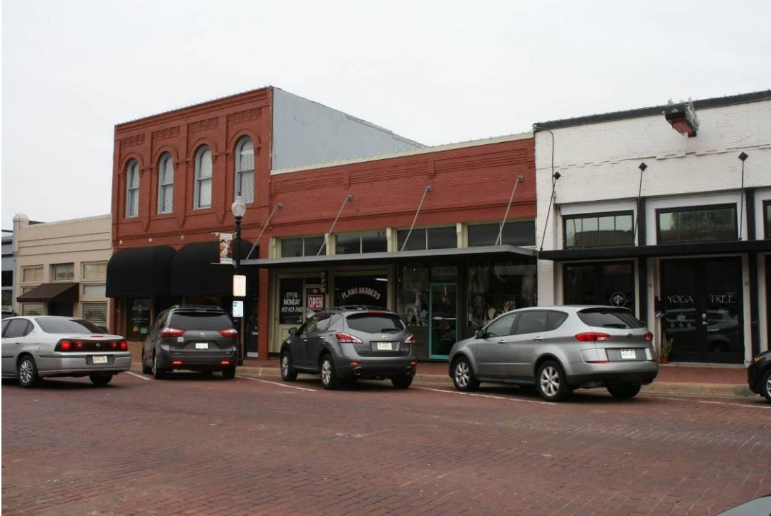
Photo 7: December 14, 2016, looking northwest at, left to right, 1027, 1029, 1031-33, and 1035 E. 15 th Street.
