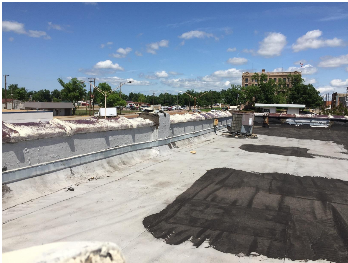
Photo 4 View of roof Camera facing East
