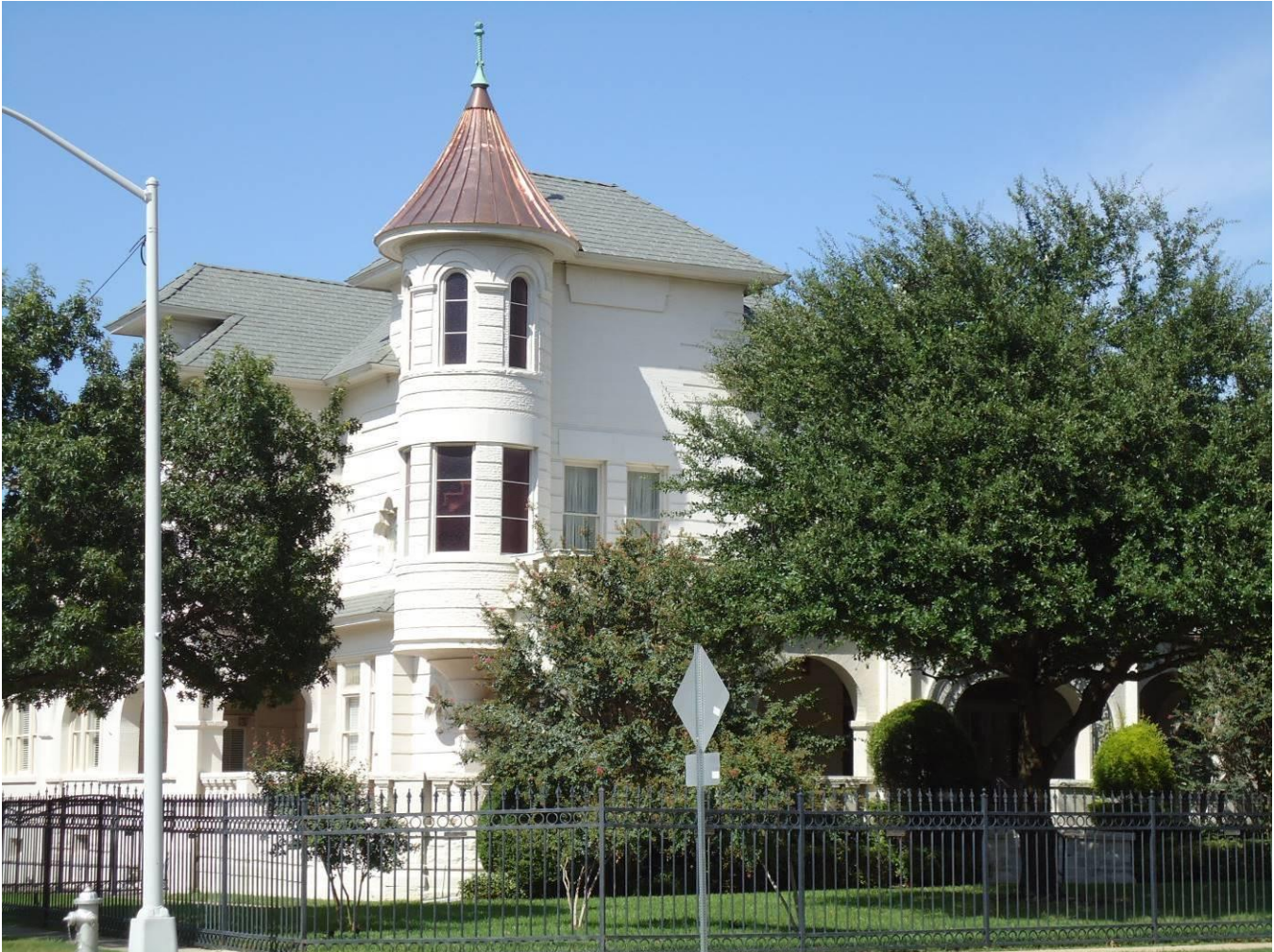
Photo 22: Margaret Meacham Hall, showing new copper and faux slate roofs, August 21, 2016, looking northeast.
