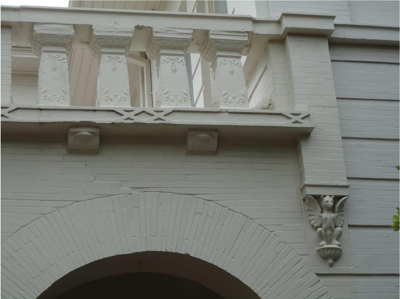
Photo 21: Margaret Meacham Hall (details, east elevation), May 25, 2016, looking west.
