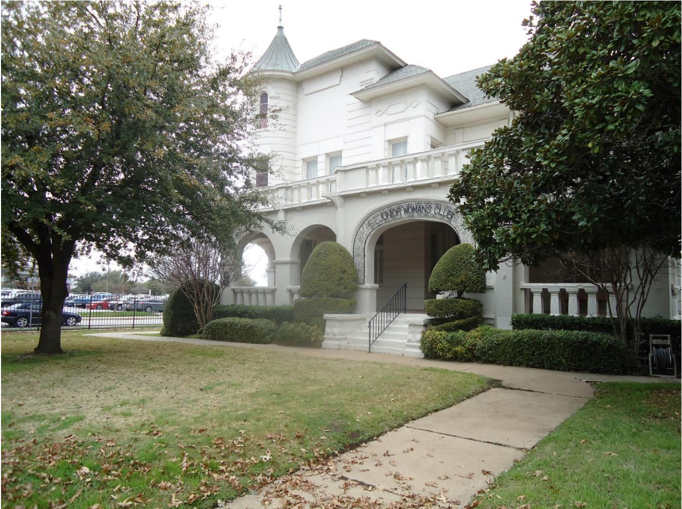
Photo 20: Margaret Meacham Hall, March 18, 2015, looking northwest.
