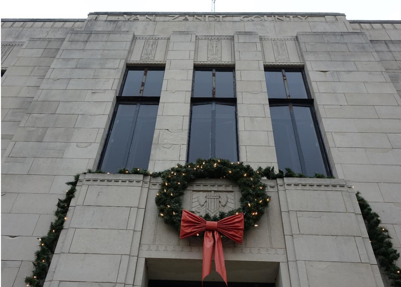
Photo 3: Frieze on north elevation. Camera facing south.
