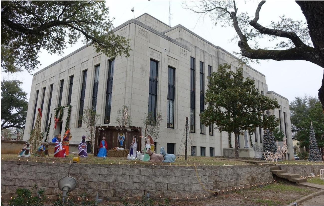
Photo 5: North and east elevations. Camera facing southwest.
