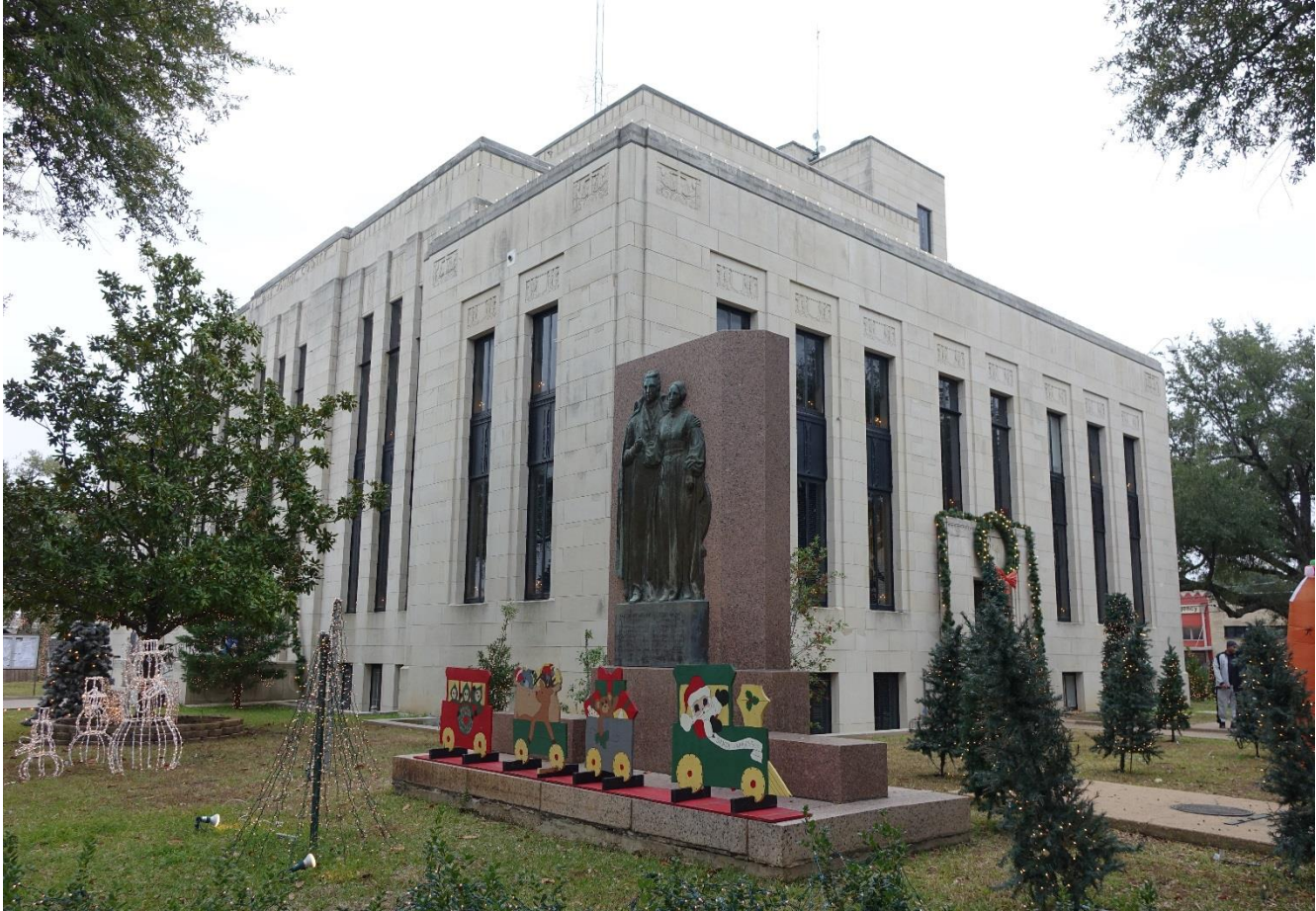
Photo 10: North and west elevations. Camera facing southeast.
