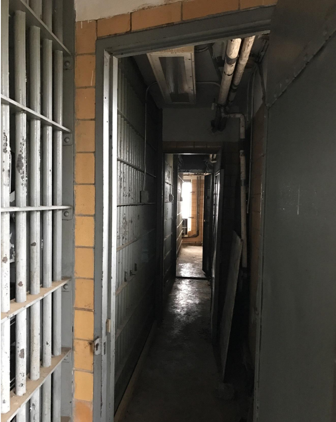
Photo 20: Corridor, fifth floor. Camera facing east.
