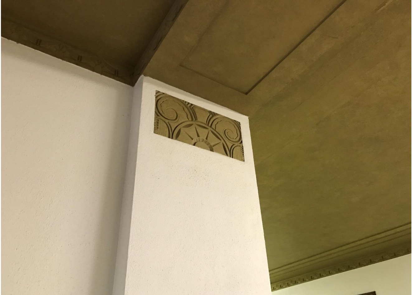
Photo 14: Coffered ceilings. Camera facing east.
