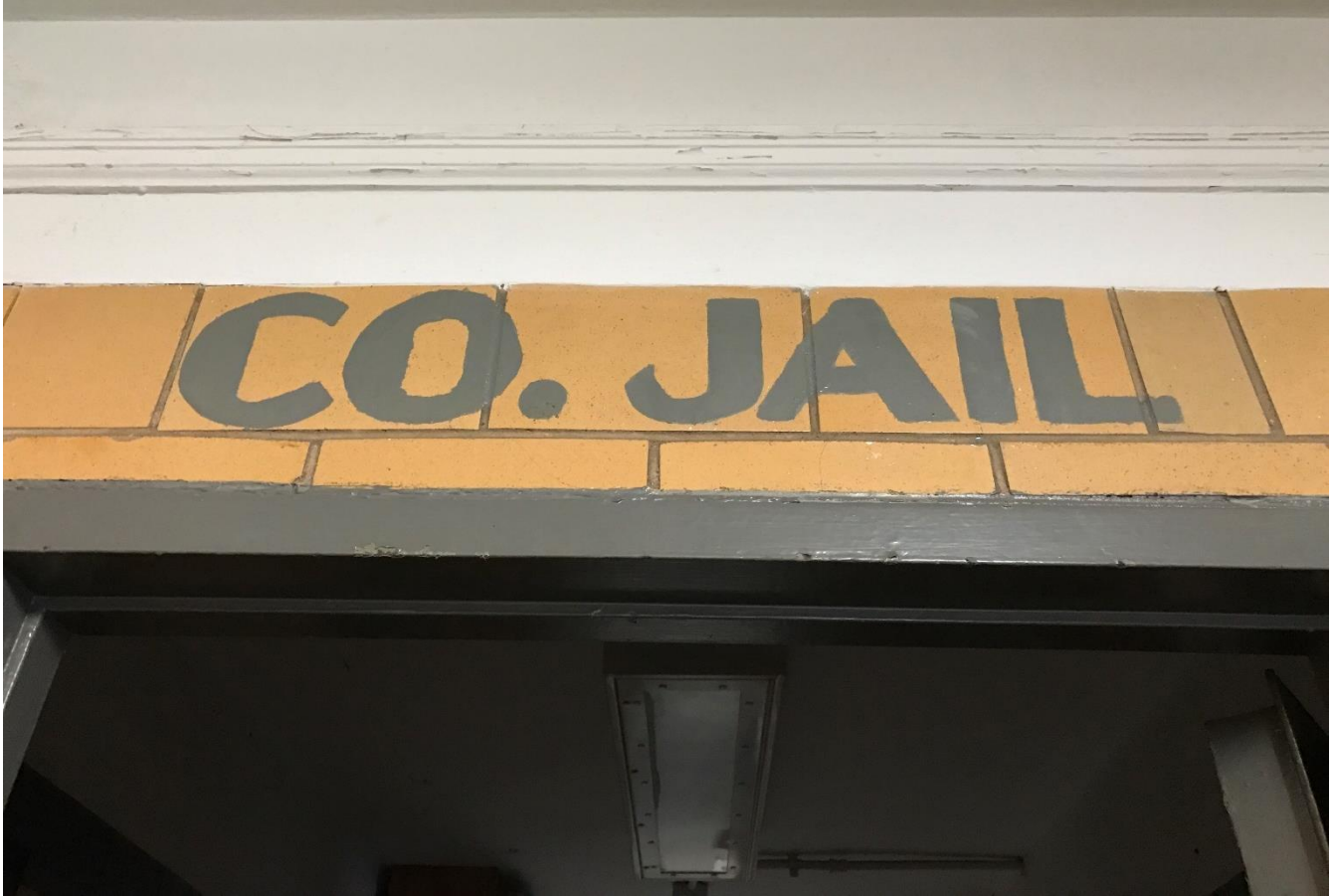
Photo 19: County jail, fifth floor. Camera facing east.
