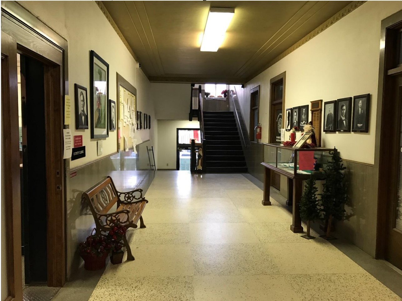
Photo 15: Second floor (main) corridor. Camera facing east.
