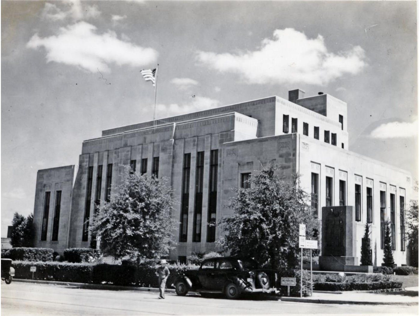
Figure 2: Van Zandt County Courthouse, ca. 1940 Photo courtesy Texas Department of Transportation
