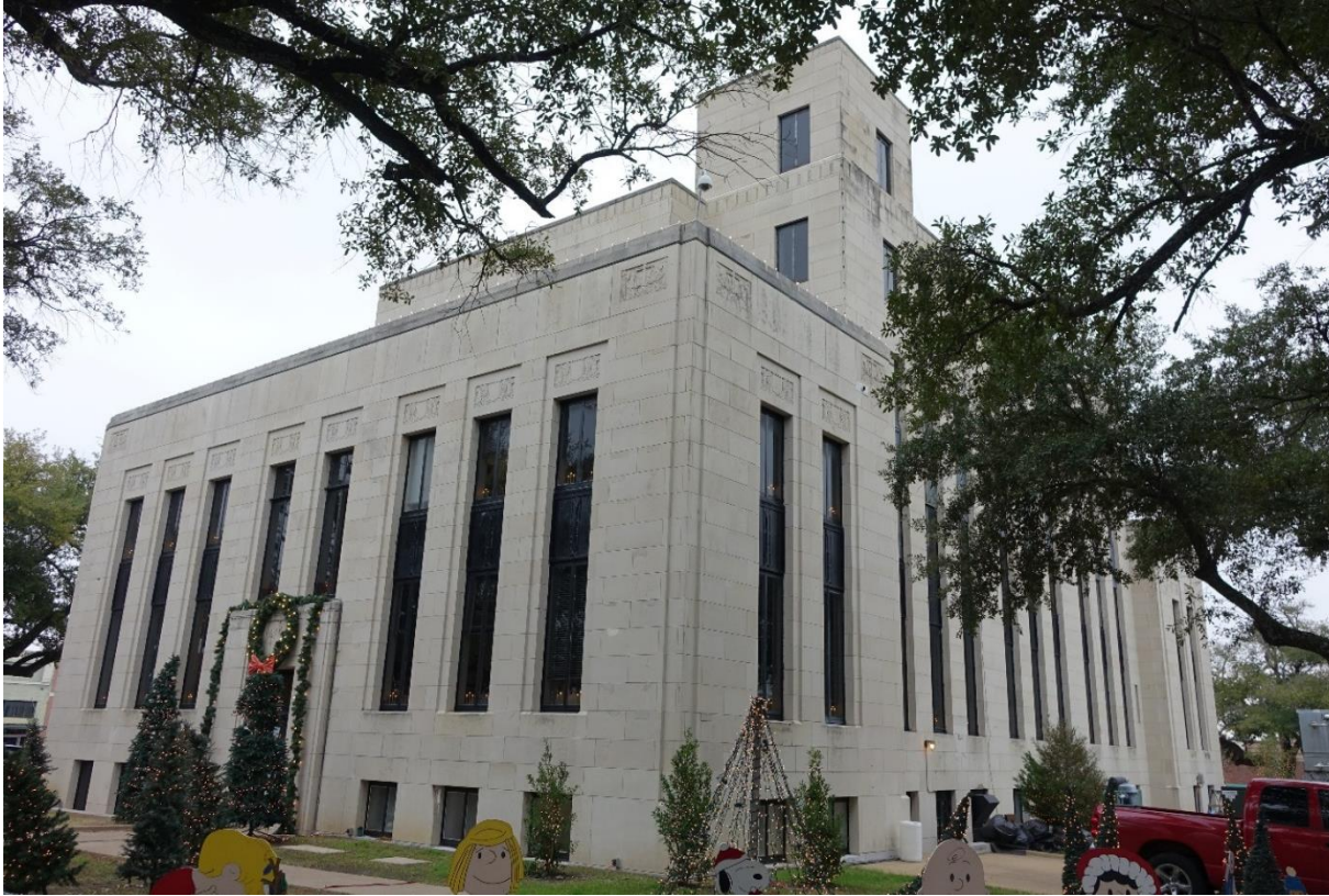
Photo 8: South and west elevations. Camera facing northeast.
