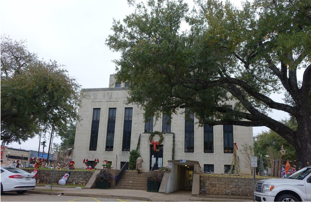
Photo 6: East elevation with ADA entrance. Camera facing west.
