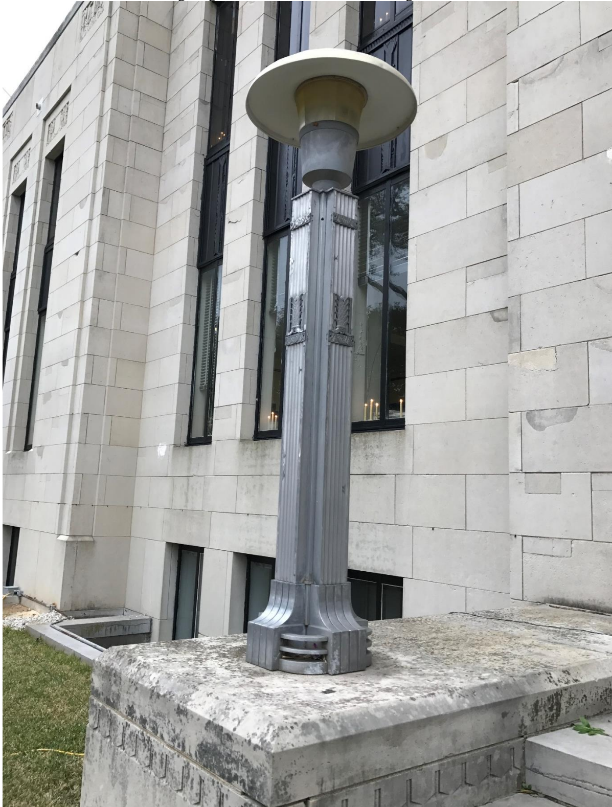
Photo 4: Art Deco exterior lighting, north elevation. Camera facing southeast.
