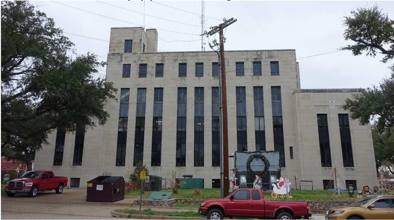
Photo 7: South elevation with utility equipment. Camera facing north.
