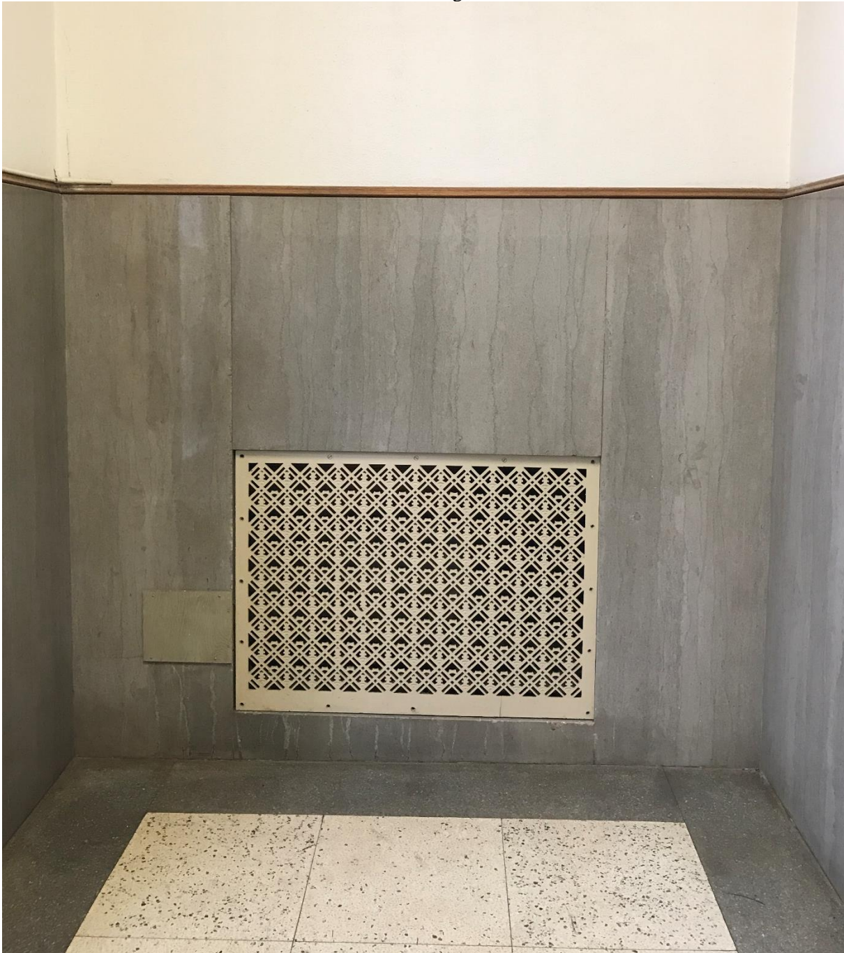
Photo 12: Marble wainscot in vestibule. Camera facing west.
