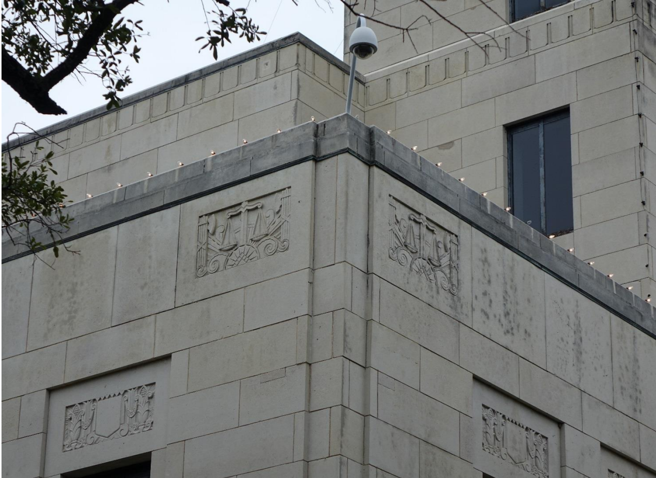
Photo 9: Decorative sculpted panels. Camera facing northeast.
