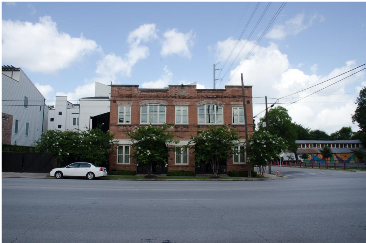
Photo 2: Primary (east) elevation. Camera facing west.
