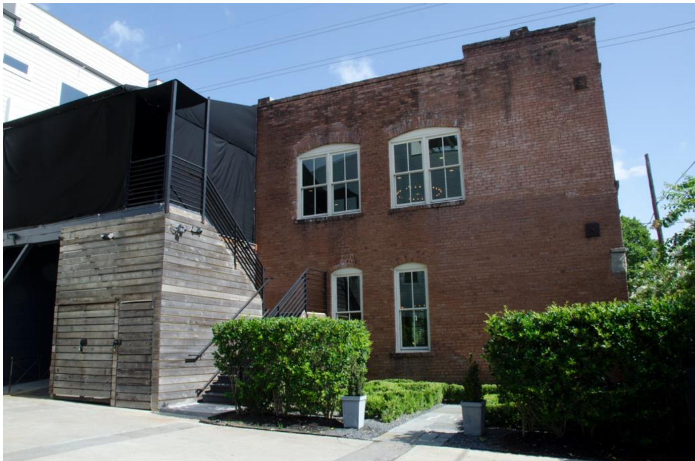
Photo 9: South elevation. Camera facing northwest.
