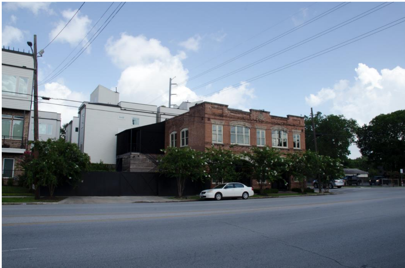
Photo 8: East & south elevations. Camera facing northwest.
