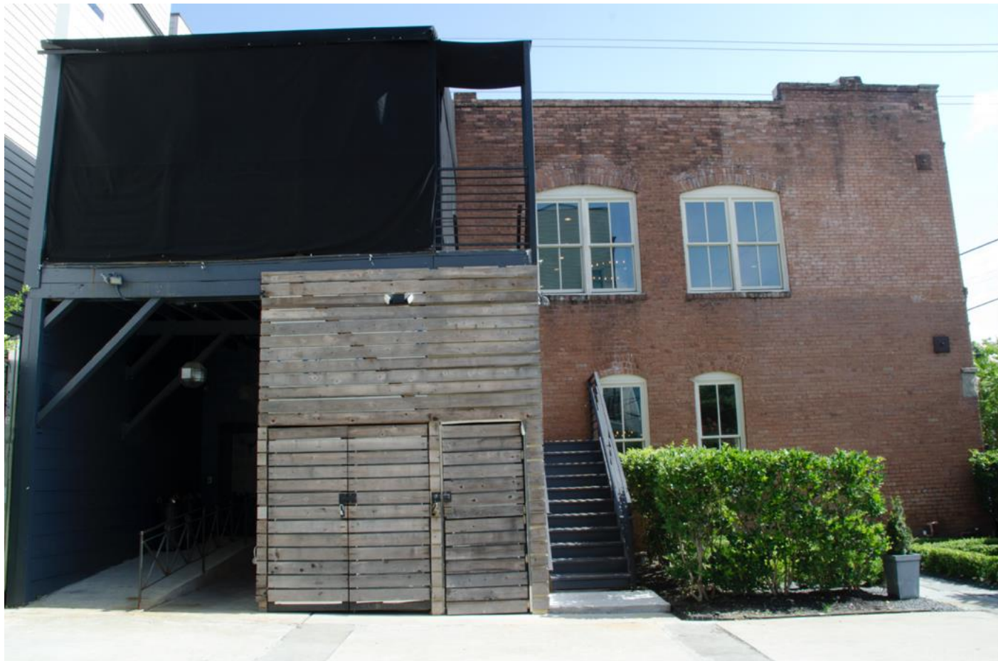
Photo 10: South elevation. Camera facing north.
