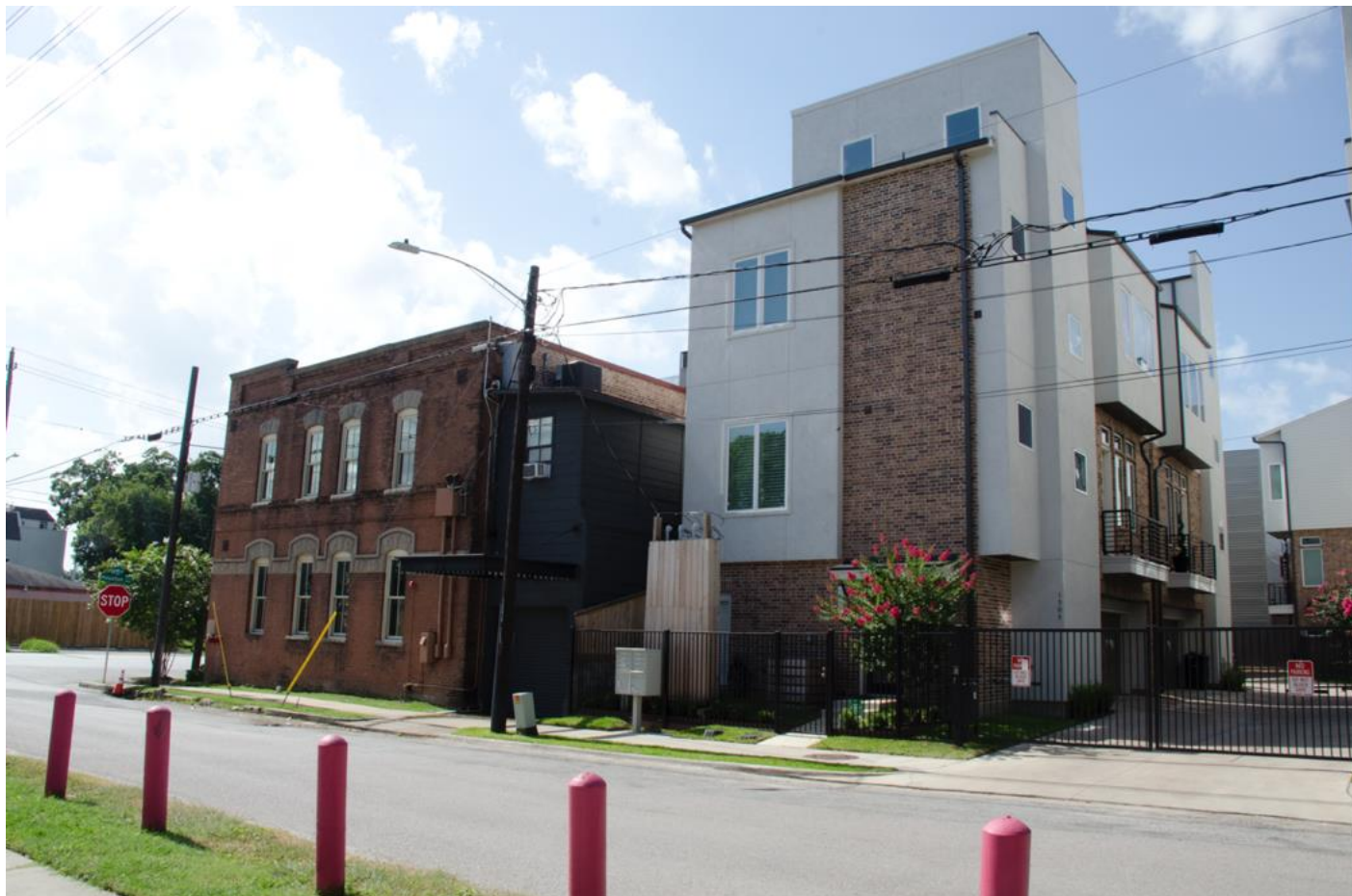
Photo 7: North & partial west elevation. Camera facing southeast.
