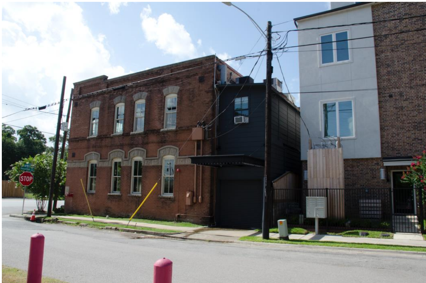
Photo 6: North & partial west elevation. Camera facing southeast.
