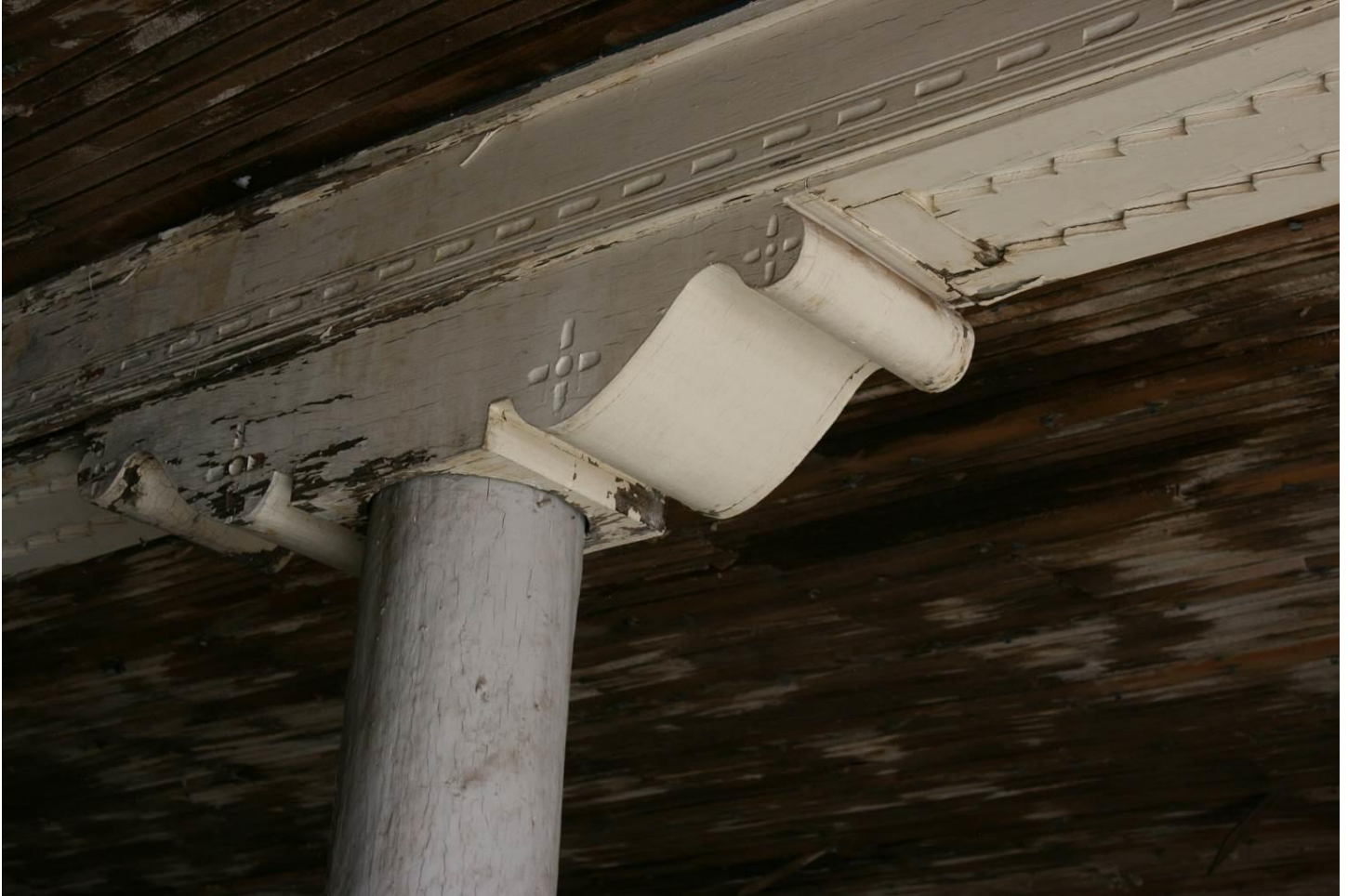
Photo 9: Carved beam and column capital.
