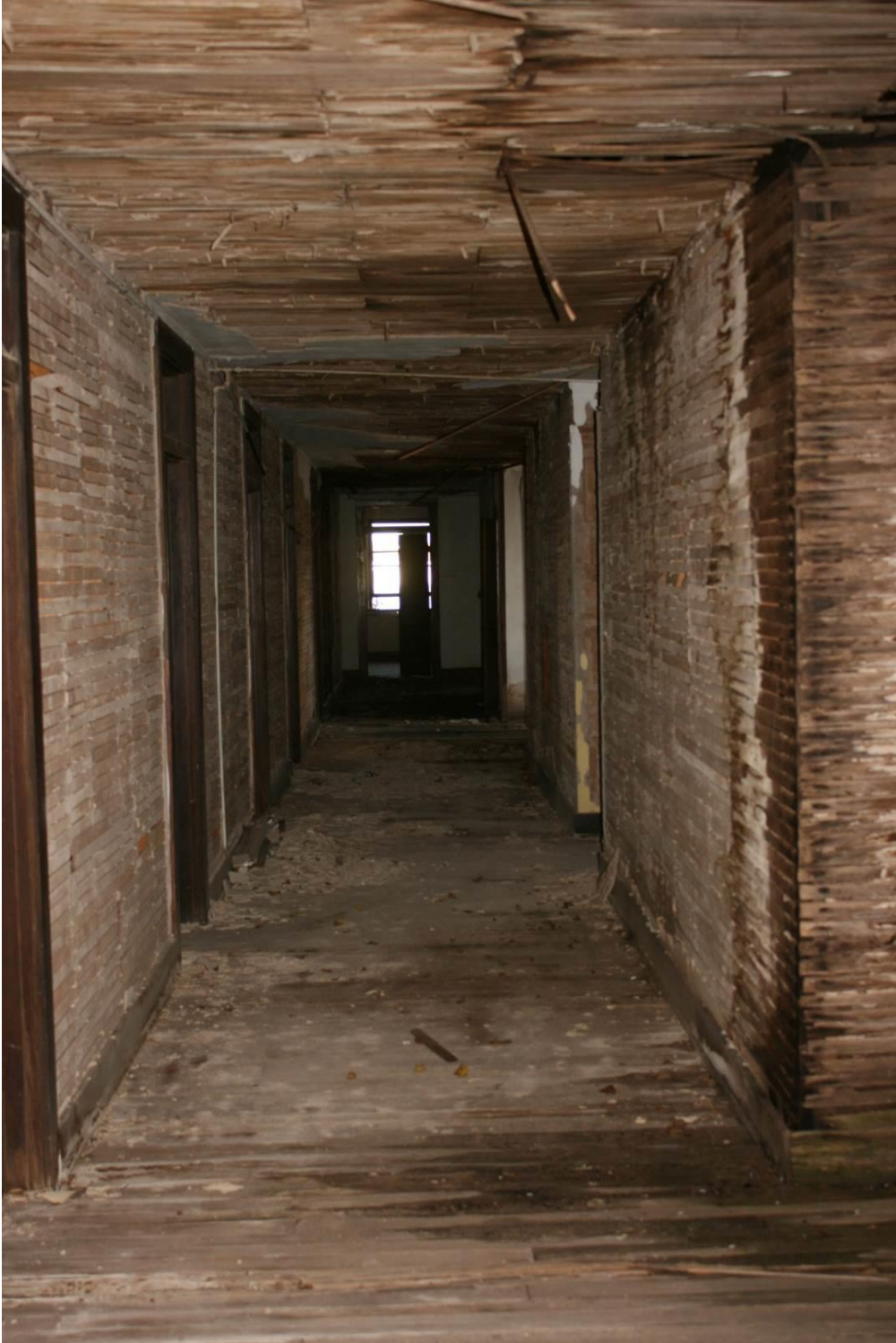
Photo 11: Second floor; East-west corridor. Camera facing east.
