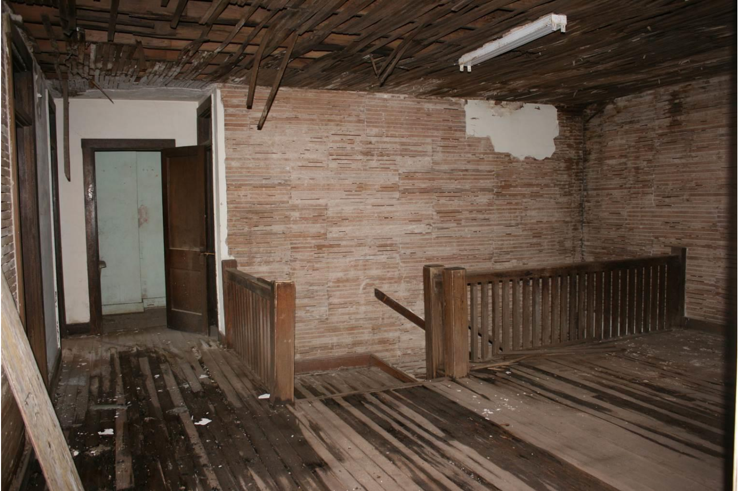
Photo 10: Second floor; landing. Camera facing north.
