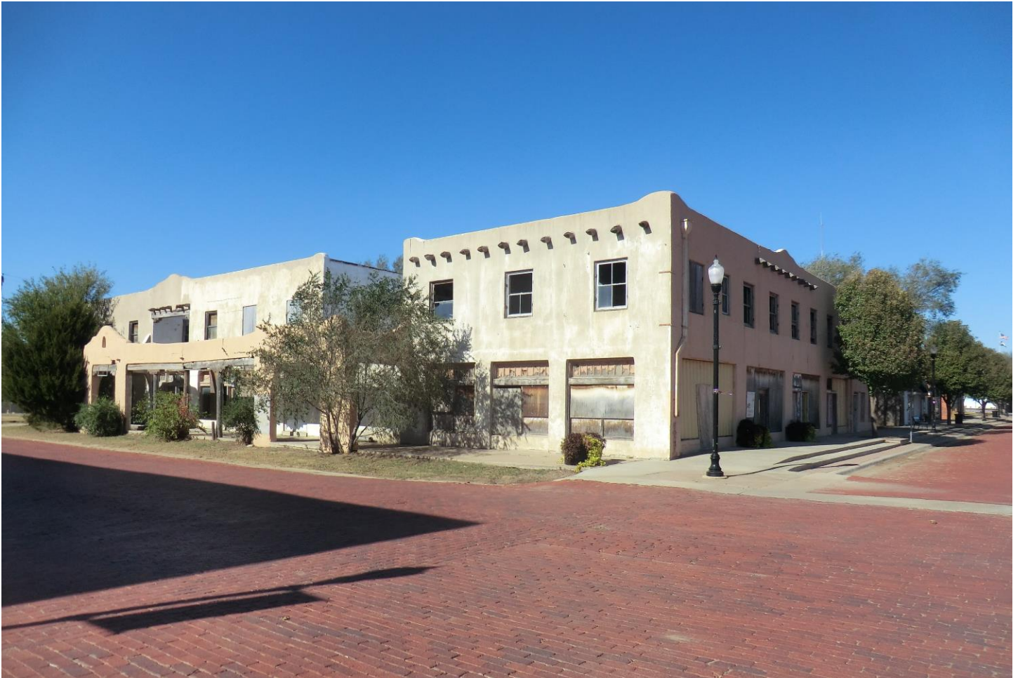
Photo 3: South and east elevation. Camera facing northwest. Photograph taken by Paul Katz November 13, 2016.
