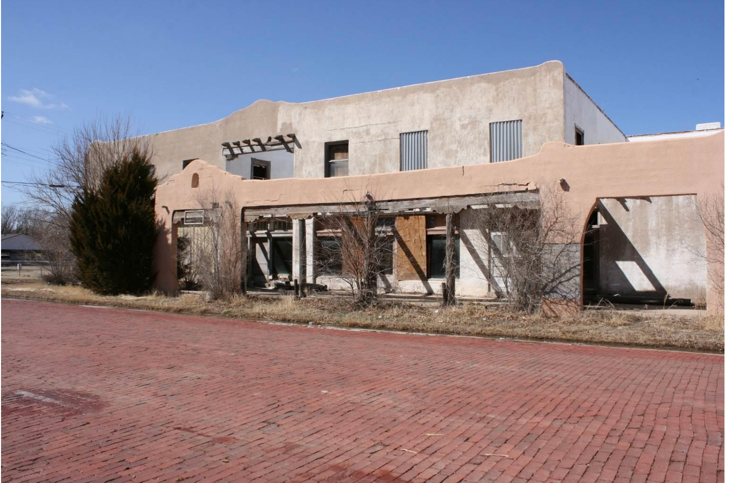
Photo 2: South elevation. Camera facing north.
