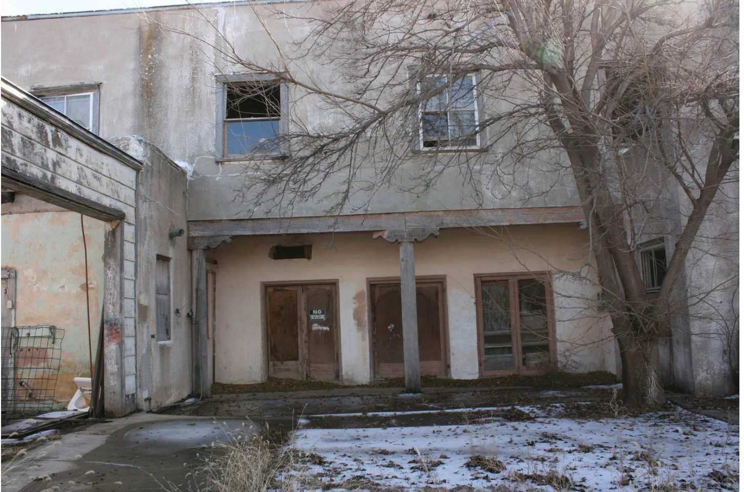
Photo 5: North elevation. Patio area on the north side. Camera facing south.
