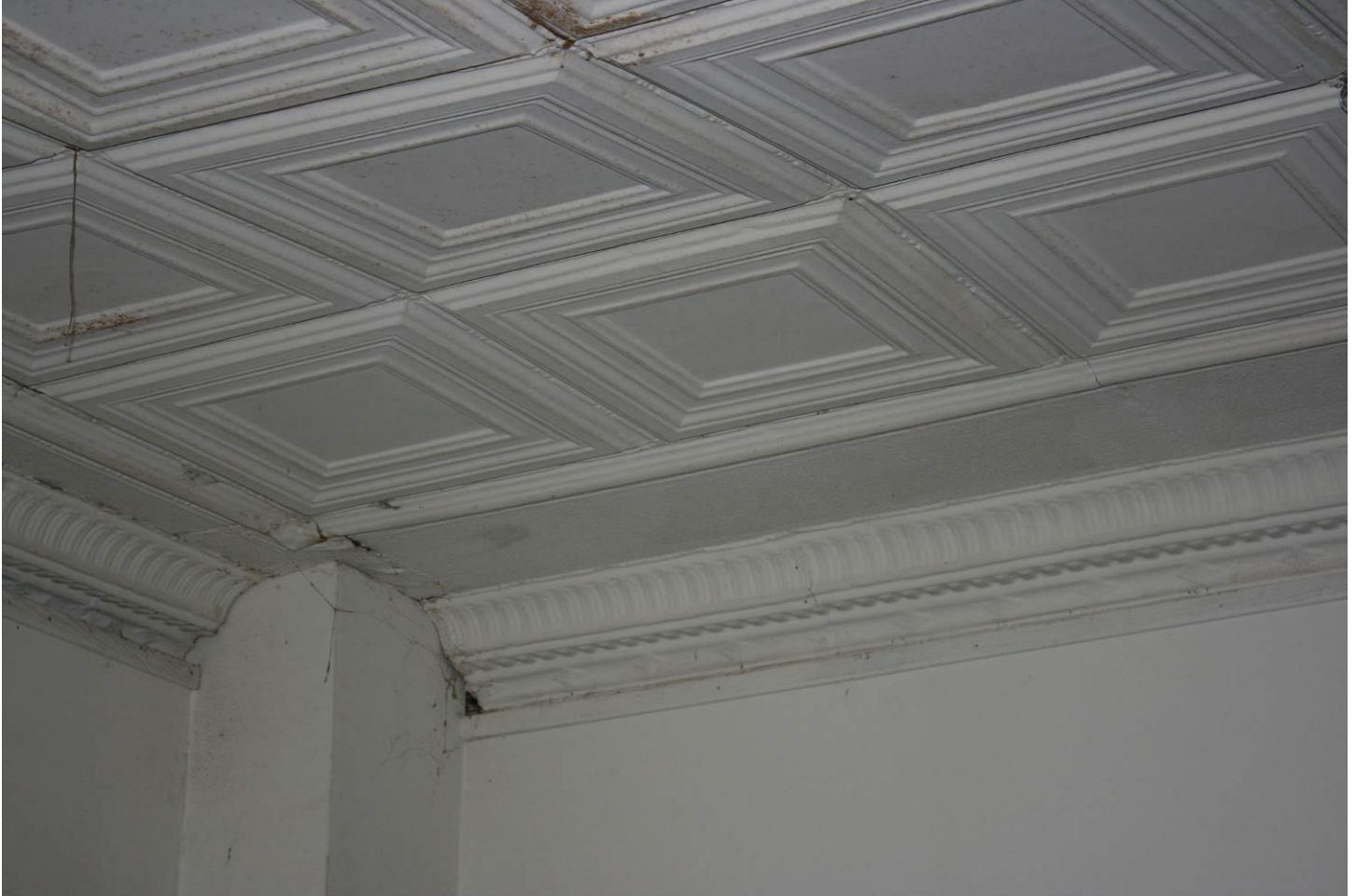
Photo 8: Pressed metal ceiling in a retail space.
