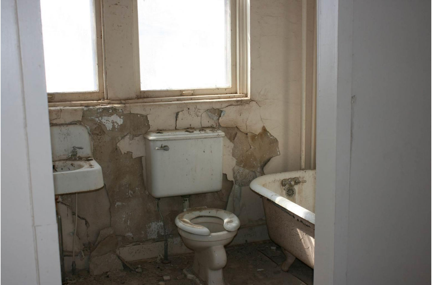
Photo 14: Second floor; private bathroom in the southwest corner room. Camera facing south.
