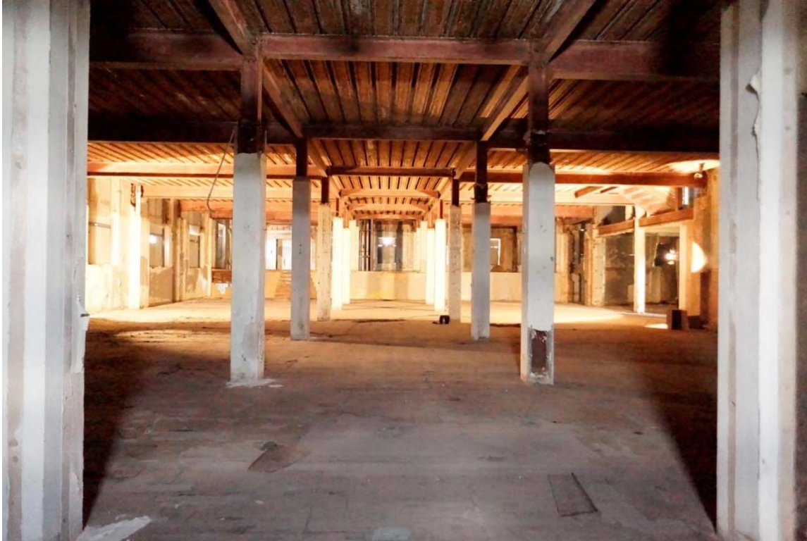
Photo 16, interior looking north, fourth floor, May 14, 2015
