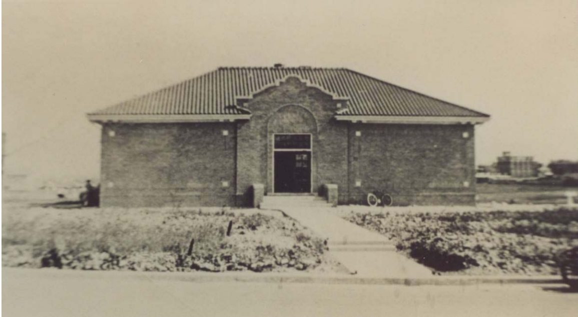
Figure 1: Lily B. Clayton Elementary School, 1922, looking at front (south) elevation. Note the Mission-shaped parapet and the lack of windows on this elevation. Courtesy Lily B. Clayton Archives.
