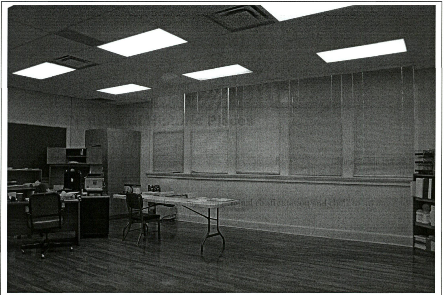
Figure 5: Celina Public School, typical classroom with original configuration and chalkboard intact (room converted to office space), camera facing west (2007).
