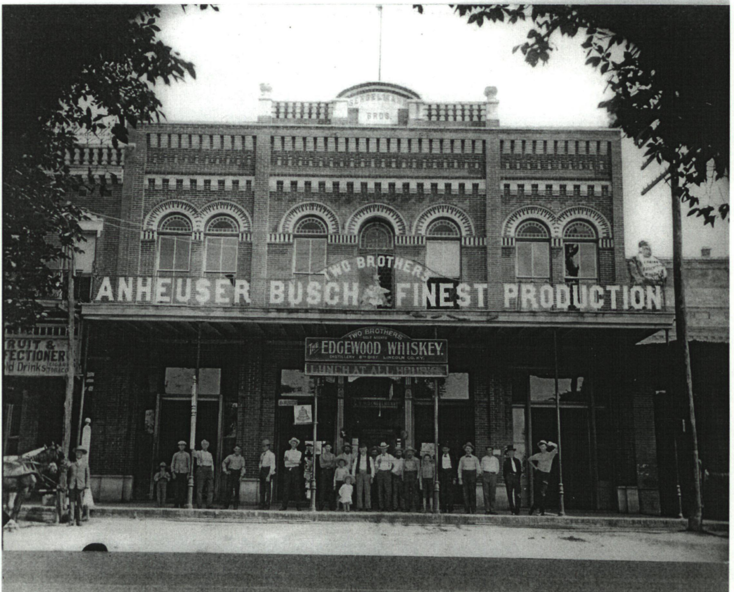
Sengelmann Hall, South façade, c1920
