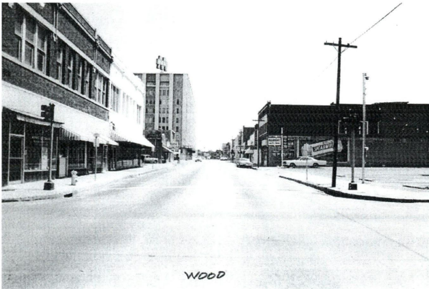
Photograph 4H: South Ervay Street from intersection at Wood Street. 400 South Ervay at left with 416, 418 and 420 marginally visible on other side of 2 nd (white) building which has been demolished. Buildings at right side of street have been demolished. Butler Building is tall building in background. Camera facing South.
