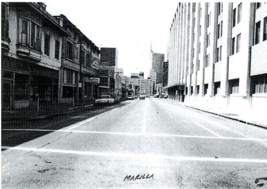
Photograph 7H: South Ervay Street from intersection at Marilla Street. Butler Building is at right; buildings at left side of street have been demolished (site of Dallas City Hall). Camera facing North.
