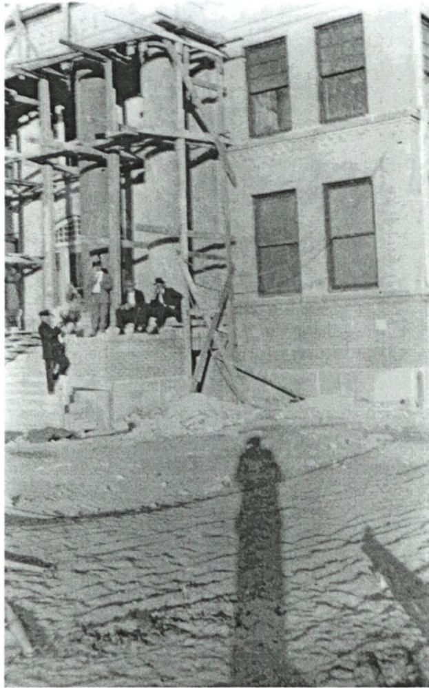
Photo 4. Lipscomb County Courthouse under construction, 1916 Photographer and date unknown (personal collection of Debby Opdyk and Jan Luna)
