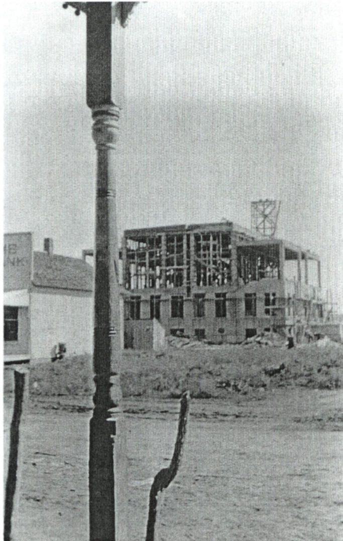
Photo 2. Lipscomb County Courthouse under construction, 1916 Photographer and date unknown (personal collection of Debby Opdyk and Jan Luna)
