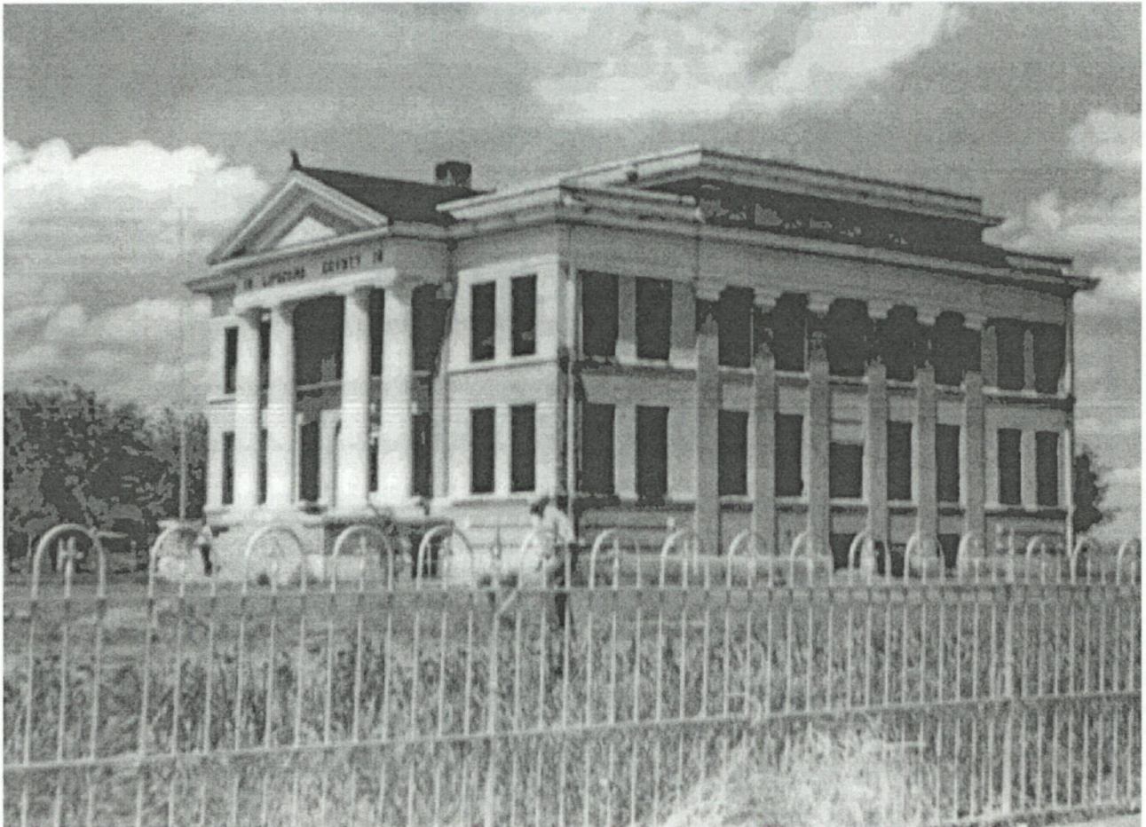
Photo 7. Lipscomb County Courthouse and iron fence (since removed) Photographer and date unknown (personal collection of Debby Opdyk and Jan Luna)
