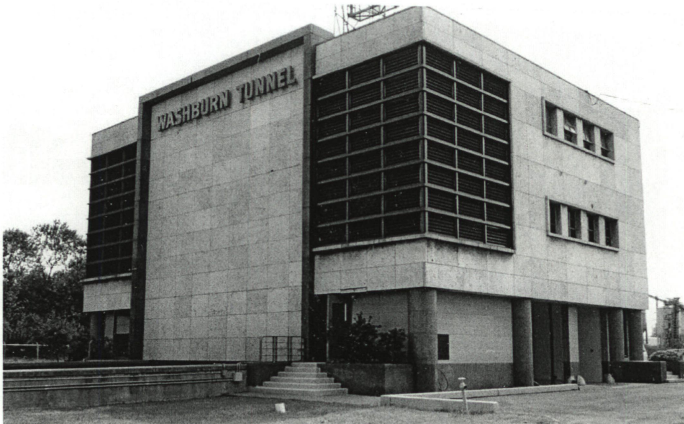
Photo 12. Washburn Tunnel, ventilation control building, 1991. These original cast stone panels remain in place under a removable slipcover of zinc currently covering all four façades. Photograph courtesy of Harris County.
