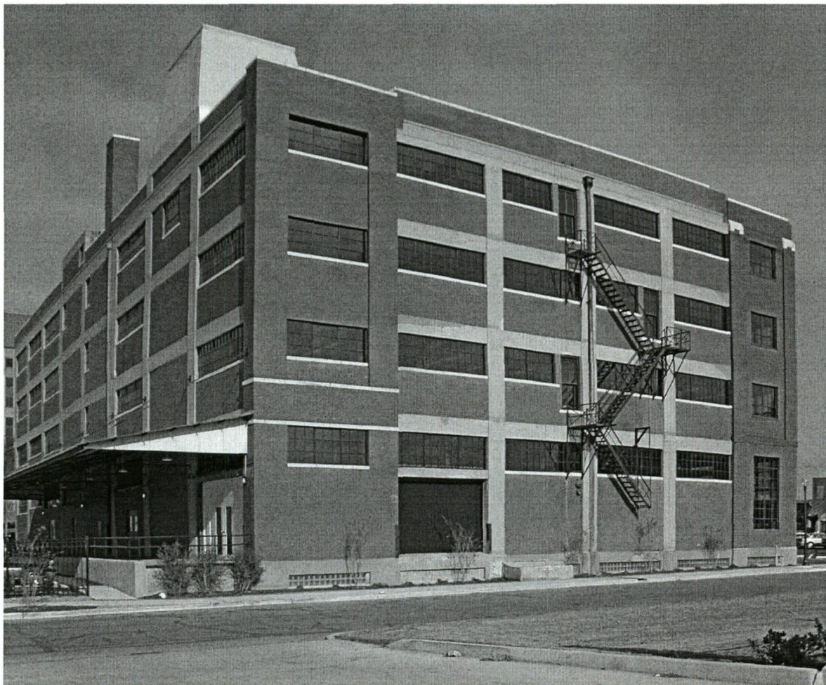
Photo 6. South elevation with former loading dock and fire escape.
