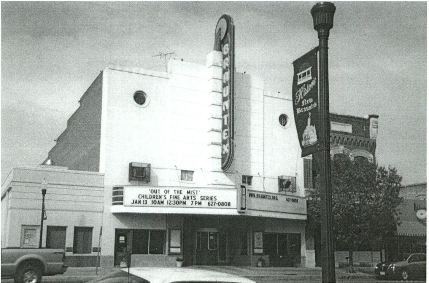
Figure 4. Brauntex Theater 2006. To the left is the non-historic addition built during renovation in 1999. To the right, the bank building shown in Figure 2.
