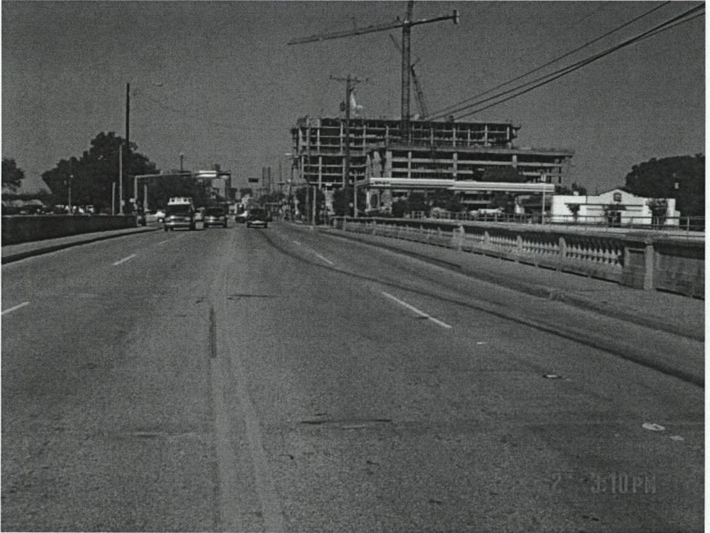
Photo 3: Roadway photo of bridge, facing north. Photo by Greg Harmon.
