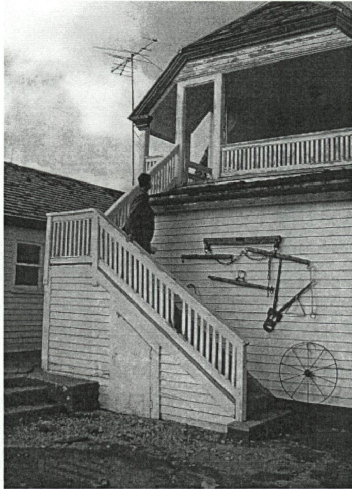
Fig. 8. Recent photograph of south side of rear stair and sleeping porch 82
