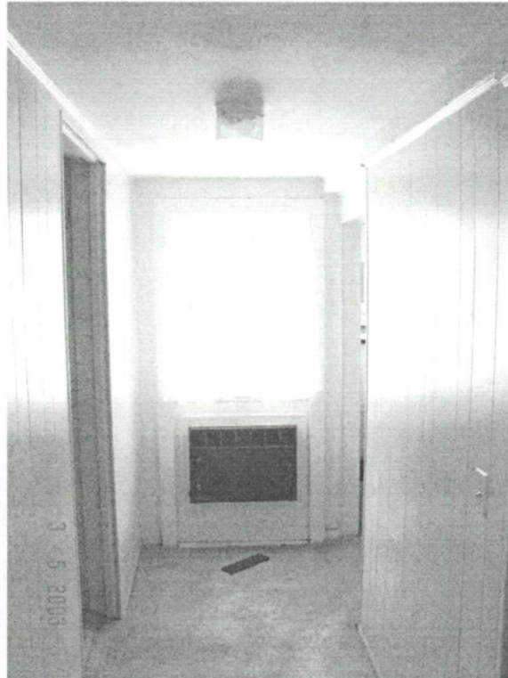
Fig. 9. Hall, looking south toward window (former doorway). Photo by author.
