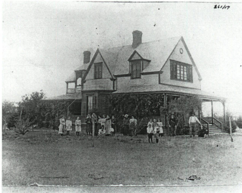
Fig. 1. Very Early Historic Photograph, estimated c. 1895. 75
