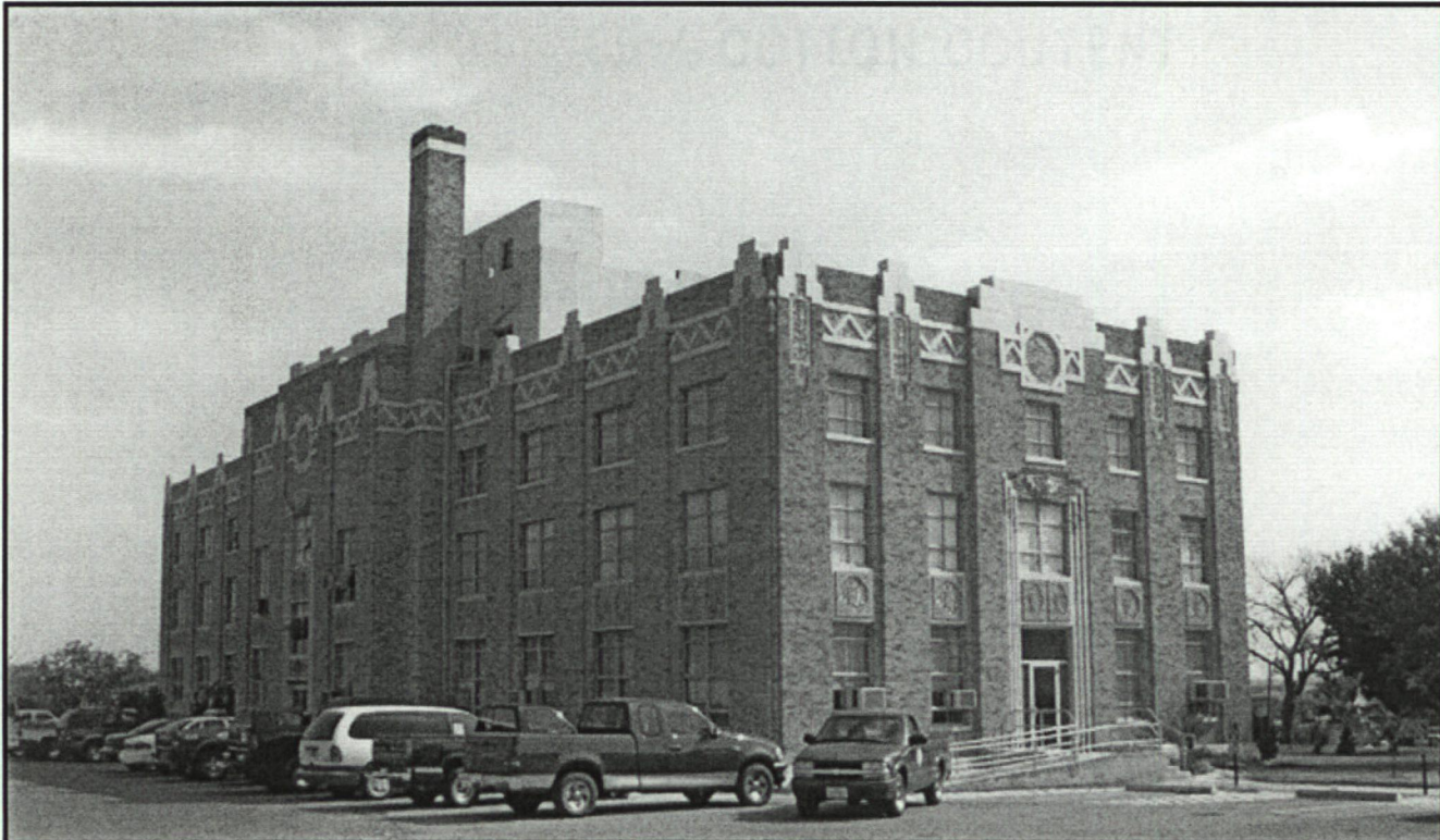
The rear (west) and south façades. The prominence of the rooftop jail and elevator penthouse are clearly shown.
