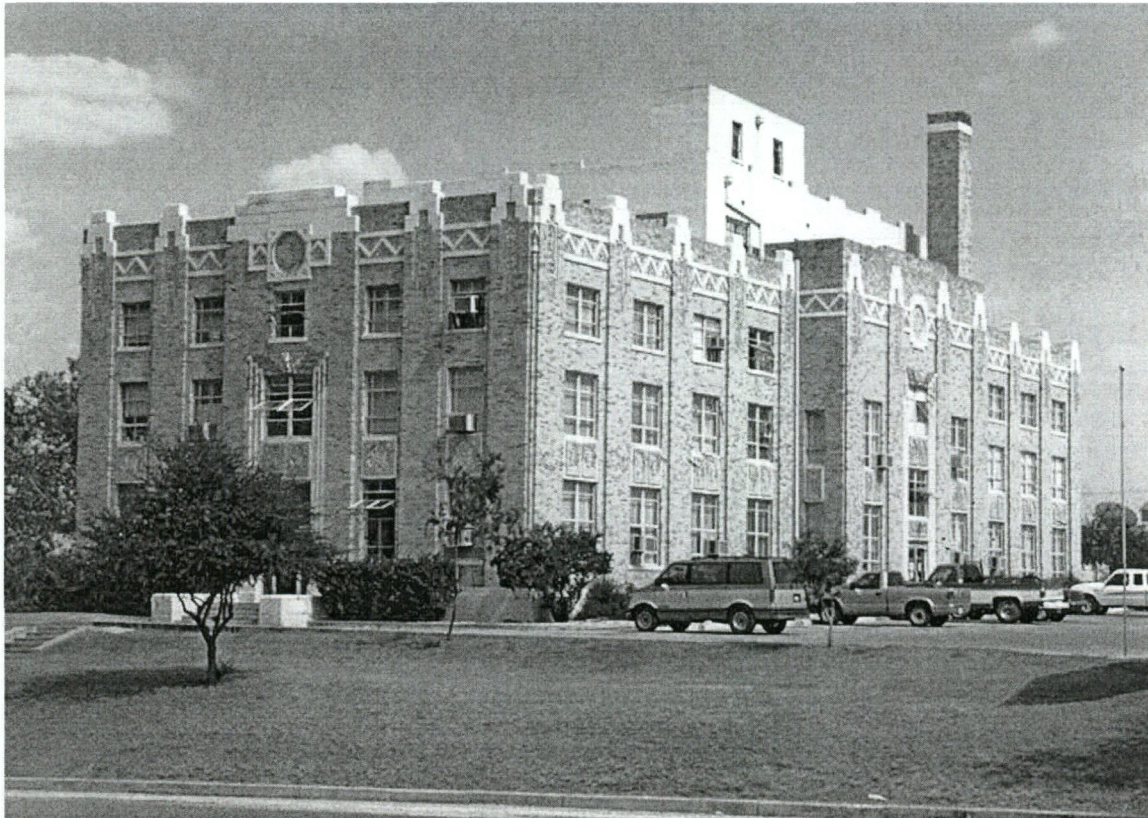
North and west elevations; parking lot on west side of building
