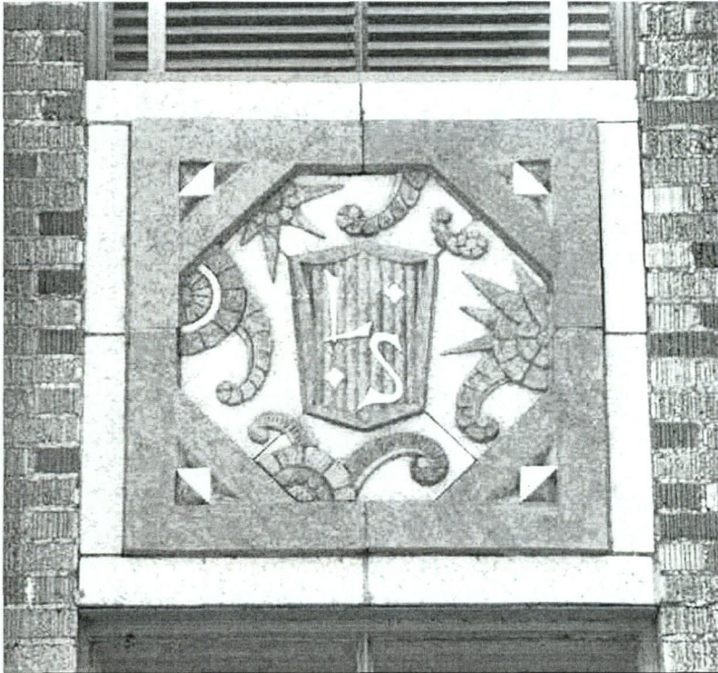
The stylized La Salle County shield of the terra cotta spandrel pieces between the first and second floors.
