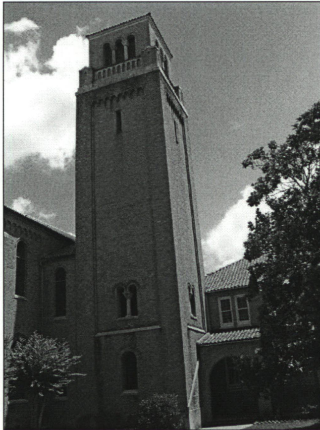
Campanile (bell tower), south oblique view.
