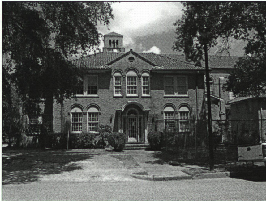
Rectory, southeast elevation.
