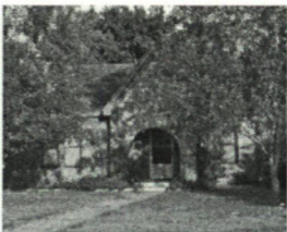
Figure 7.26. 1324 St. Marie Camera Facing East
