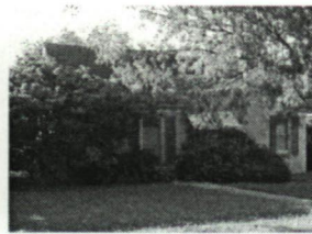
Figure 7.28. 1327 St. Marie Camera Facing Northwest
