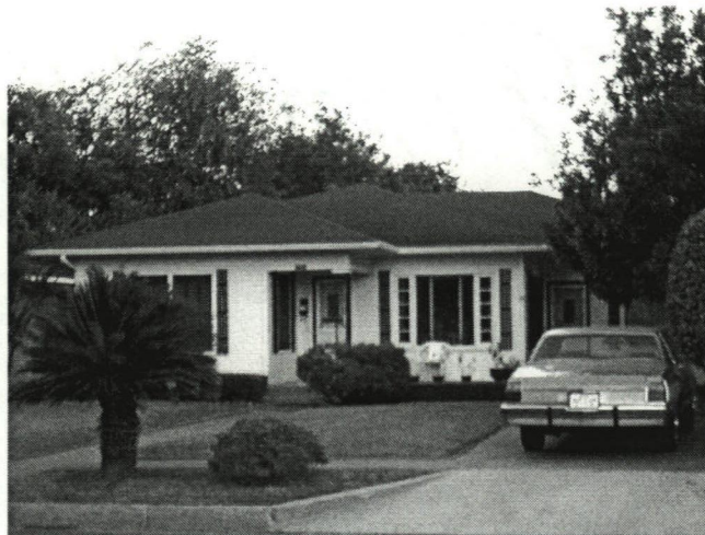
Figure 8.4. Ramiro Tijerina House. 1314 Francisco. Camera Facing East.
