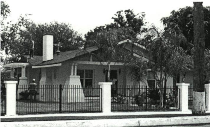
Figure 7.8. 1524 Doherty. Strickland House, 1914. Camera Facing Southwest.
