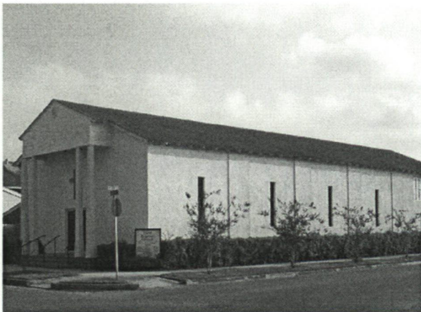
Figure 7.13. First Baptist Church. 1300 Doherty. Camera Facing Northeast.
