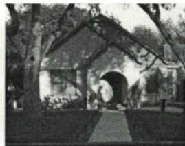
Figure 7.27. 1326 St. Marie Camera Facing East
