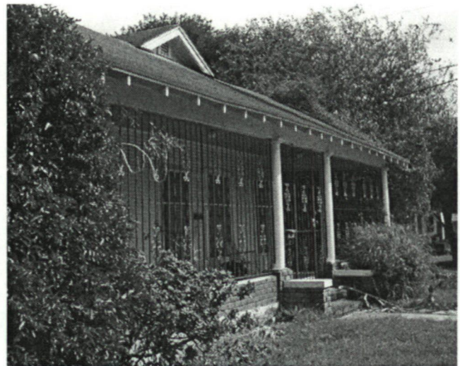
Figure 7.6. 309 E. 12 th Street. Camera Facing Southeast.
