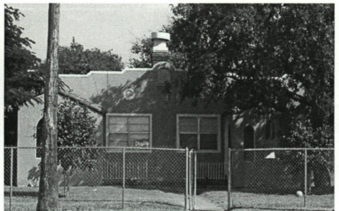
Figure 7.9. 1406-1408 Francisco. U-shaped Duplex. Camera Facing East.
