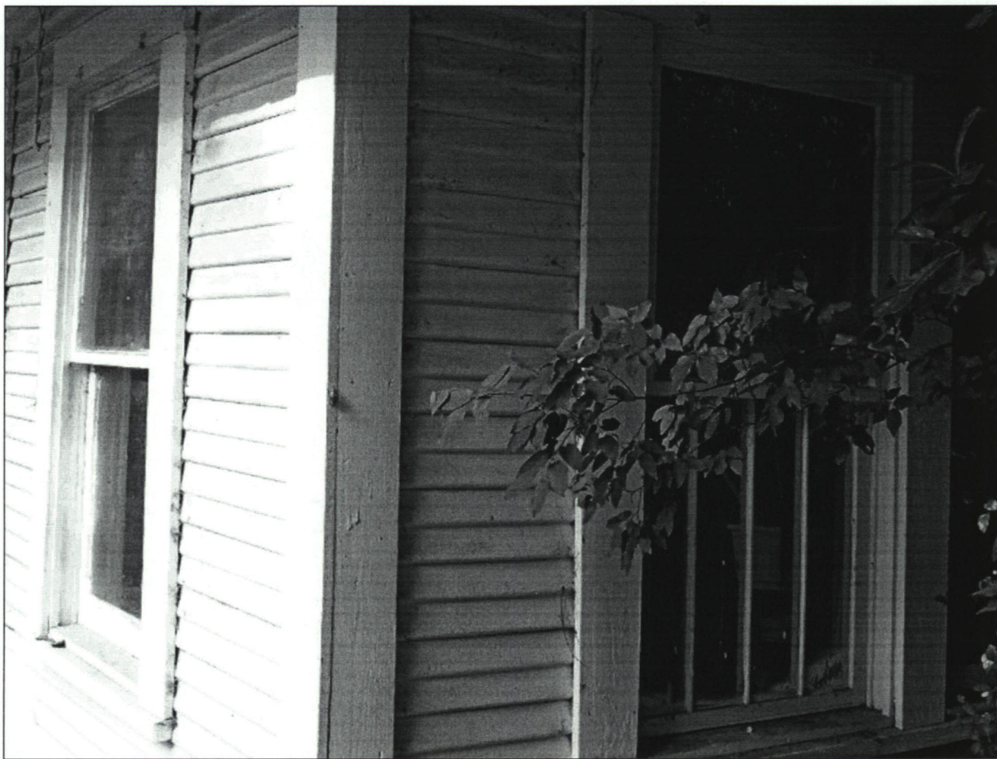
Figure 5. Canary House, northwest oblique detail.
