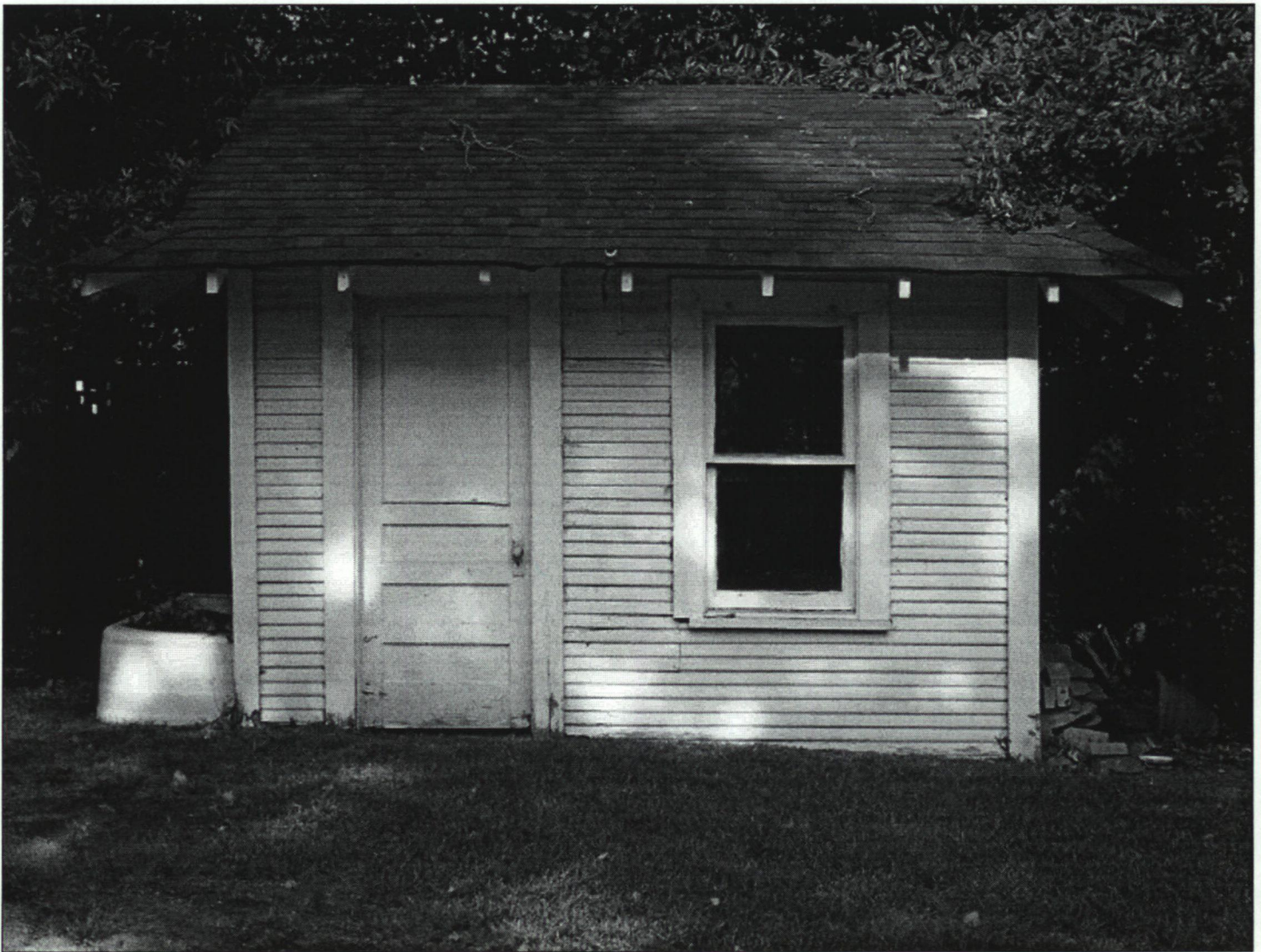
Figure 4. Canary house, north elevation.
