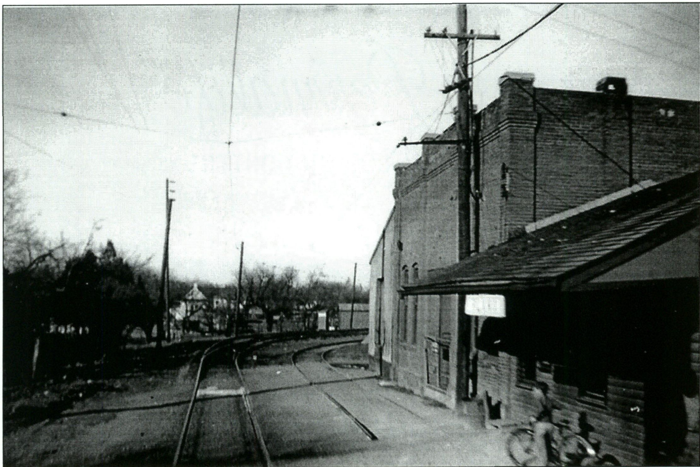
Figure 2. West elevation of Plano interurban station, circa 1930. Camera facing north.
