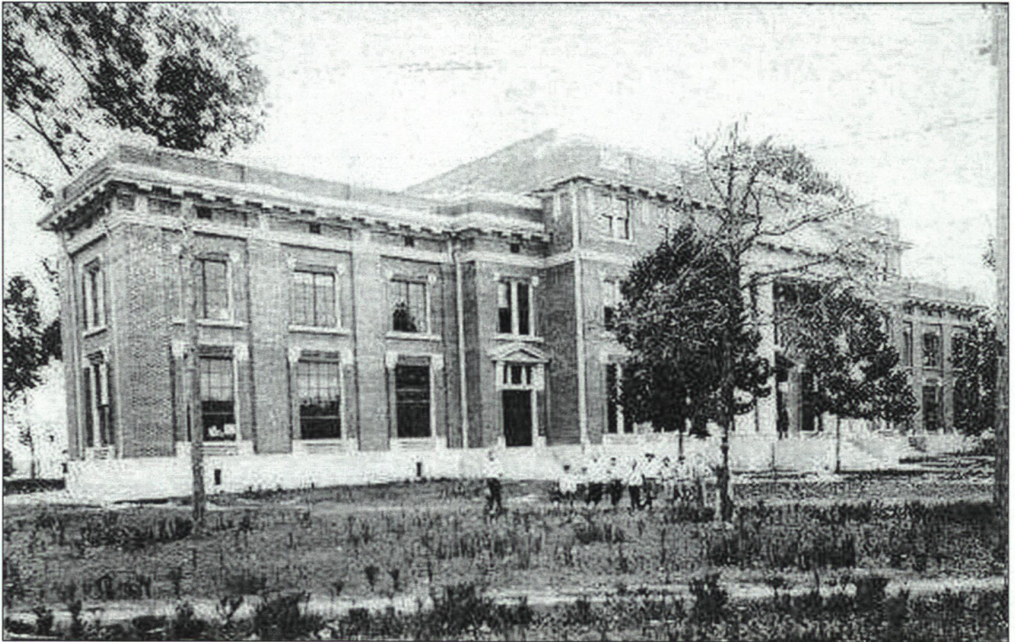
Figure 1. Trinity County Courthouse, 1917. Source: Trinity County Historical Commission.
