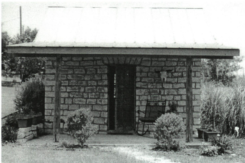
Figure 1: Creamery (West elevation, camera facing east)
