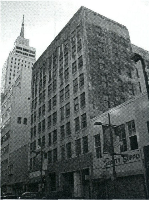
Sumpter Building (1913) 1604 Main Street
