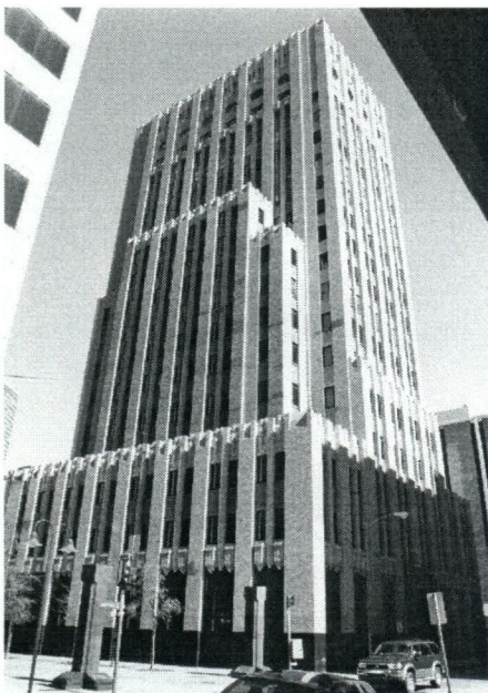
Dallas Power and Light Building (1931) 1506 Commerce Street
