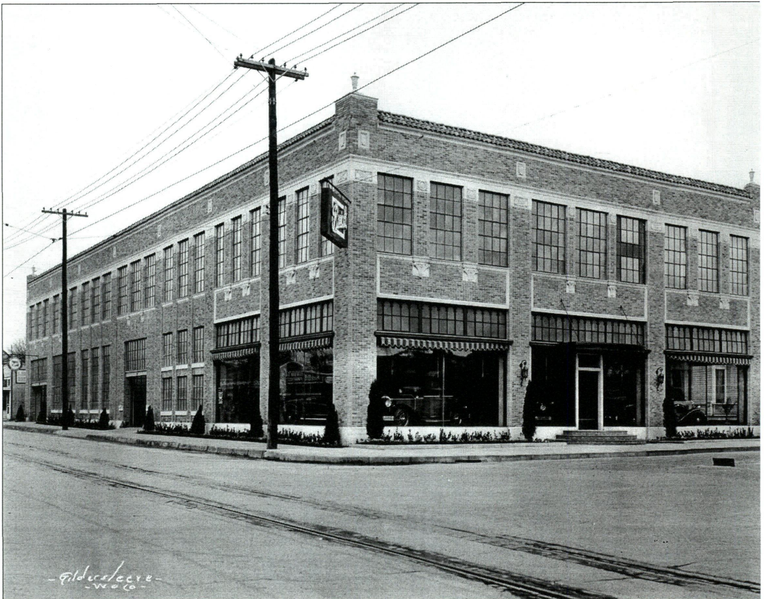
Figure 1. McDermott Motors Building, c. 1928, view from southwest. Photocopy from owner's files.
