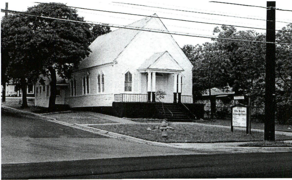
Photo #4 Church at 1100 E. 12 th Street
