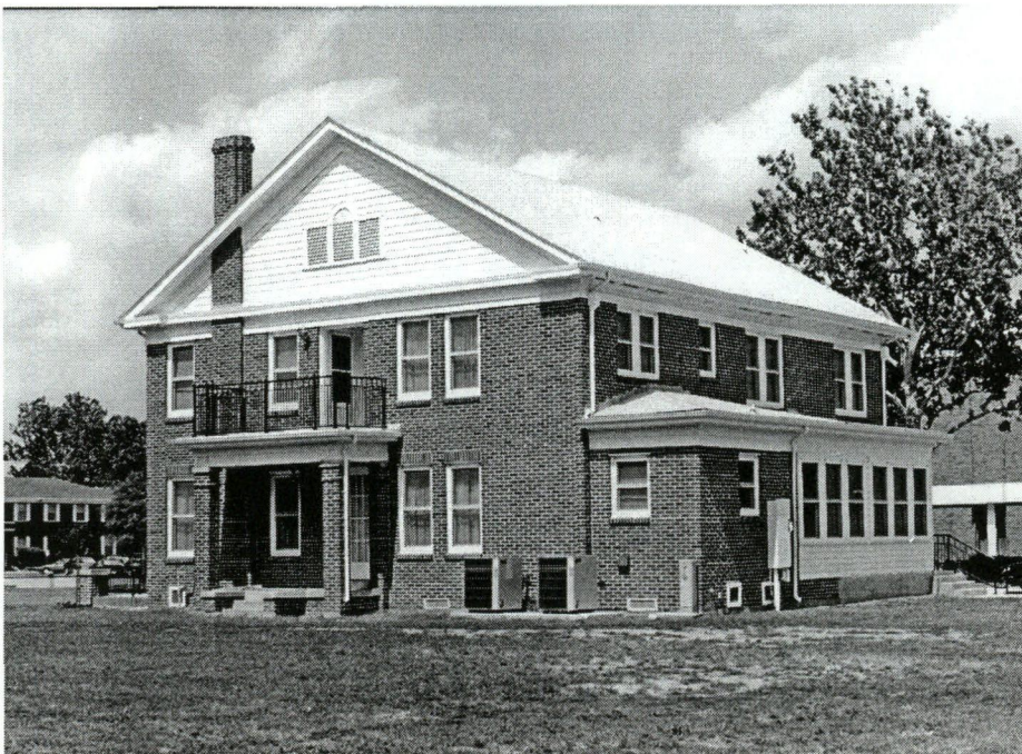
Figure 7-5. South and west facades.
