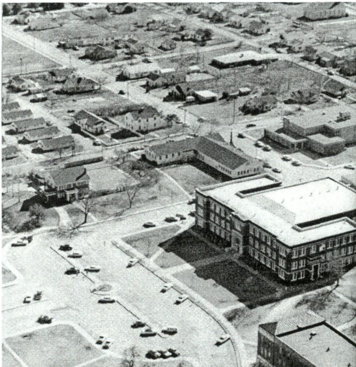
Figure 8-3. Aerial view, 1960. President's House, left center.
