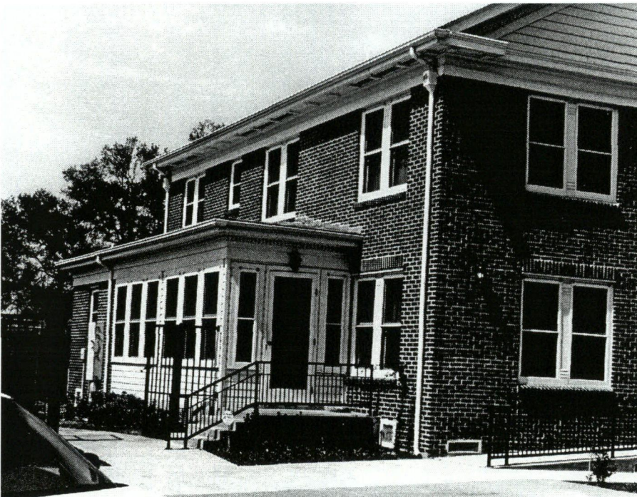
Figure 7-6. Added porch on south façade.
