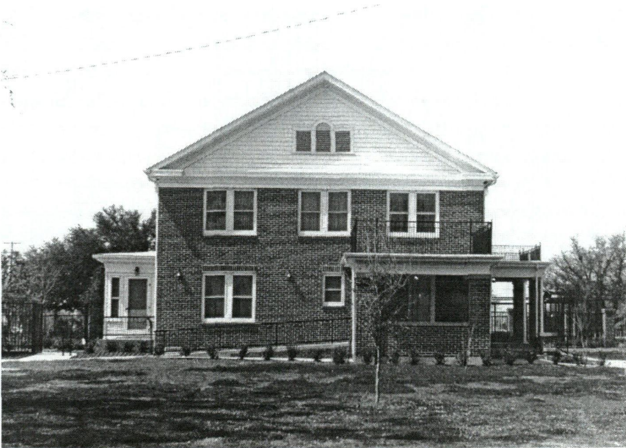
Figure 7-4. East façade with porte cochere.
