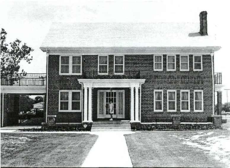
Figure 7-2. Primary (north) façade in 1996. Photographer unknown
